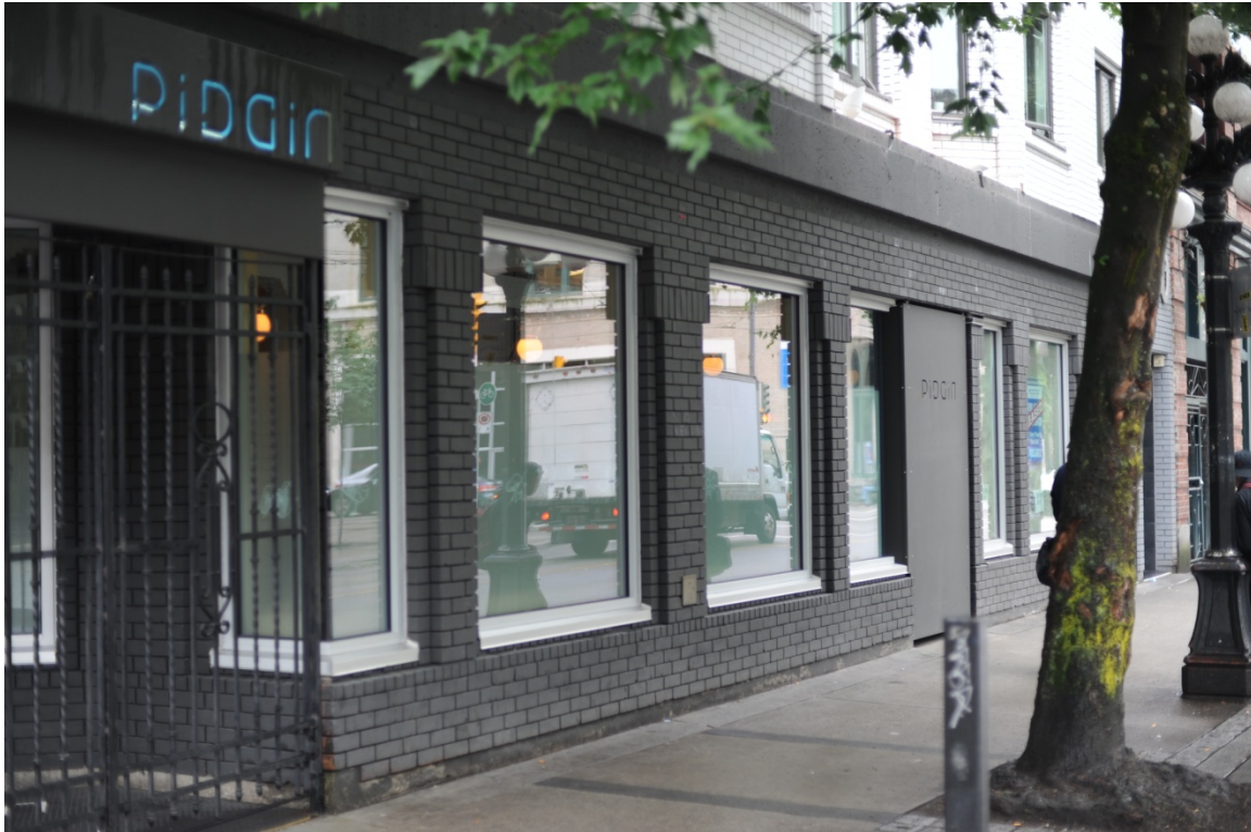
Figure 4: PiDGin. The lower two-thirds of the window are now etched a translucent white, yet when the restaurant first opened, these windows provided an unobstructed view of Pigeon Park.
