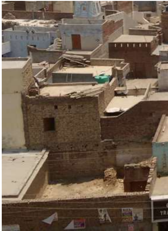
Figure 4.3: Rooftop with a Green Rooftop Water Tank, Punjab, photo taken by author May 2015
