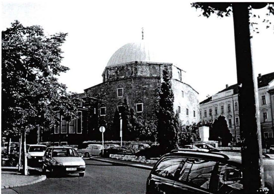
Figure 48: Semi-circular addition that replaced the original entrance and portico of the Mosque of Gazi Kasım Pasha.
