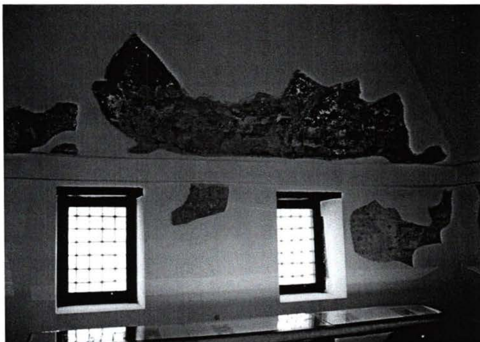
Figure 154: Upper level with the windows of the Koran school.
