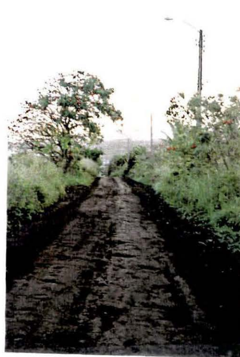
Plate 44 Some roads in Hangaroa remain unpaved and are difficult to travel. Within the next five years, all urban roads are to be paved
