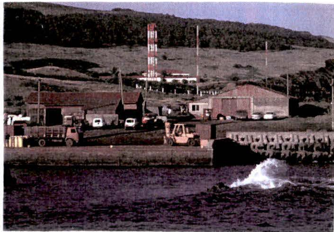
Plate 35 Supplies are unloaded onto trucks which then deliver supplies to businesses in Hangarua
