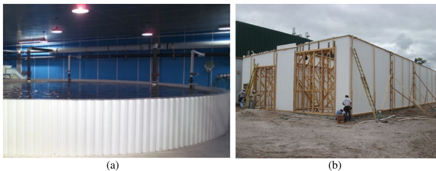
FIG. 2 SIP systems: (a) aquaculture tank; (b) wall during construction [2].
