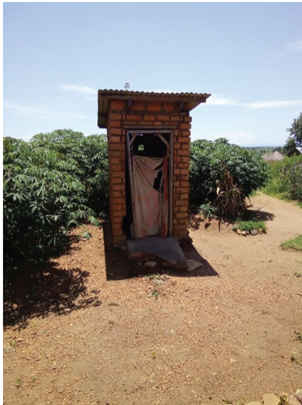
Figure 4. “You find most construct these toilets and the washrooms with unburnt bricks, so when there is too much rain . . . some of them are collapsing” (women key informant in sexual and reproductive health).
