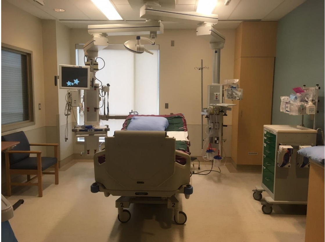
Figure 4.1: Layout of a patient room in Site A ICU (Zone 1), including bed, two booms, cardiac monitoring, and equipment cart. ICU rooms at Site B are a similar size and contain similar equipment.
