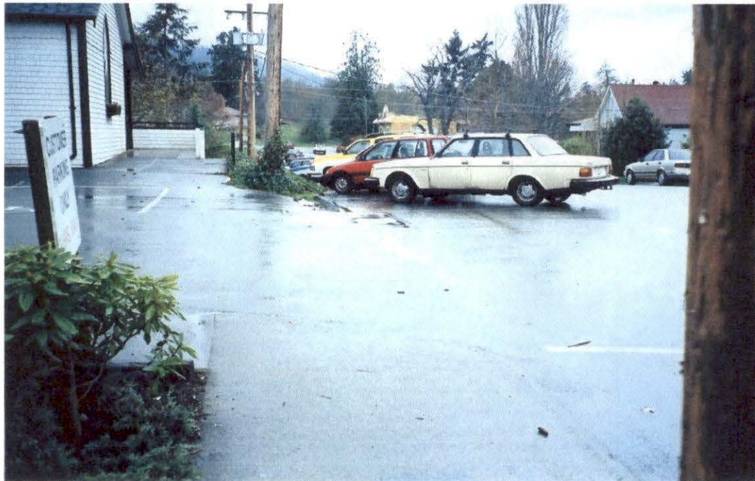
f) An illustration of a sidewalk in the core area that ends leaving pedestrians to walk on the road between parked vehicles and oncoming traffic.
