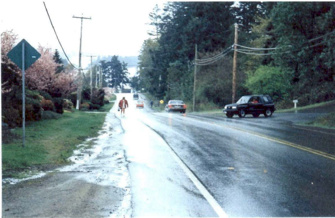
c) A pedestrian walking along the shoulder of Lower Ganges Road not only has to navigate puddles and potholes but must also watch for vehicular traffic. The shoulder in this location is about 2.5 feet in width.
