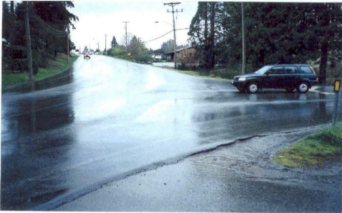
g) The intersection of Upper Ganges and Lower Ganges Roads was identified as hazardous because of the size of the intersection, the lack of vehicular control, and no crosswalk.
