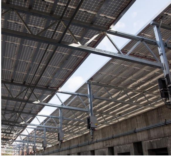
(a) Roof truss at T Rowe Price Parking Garage Baltimore, MD, United States
