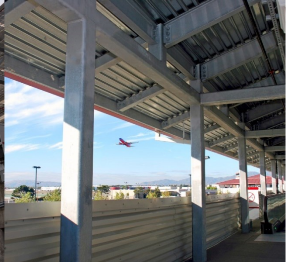
(b) Elevated pedestrian bridge at Bob Hope Airport Burbank, CA, United States
