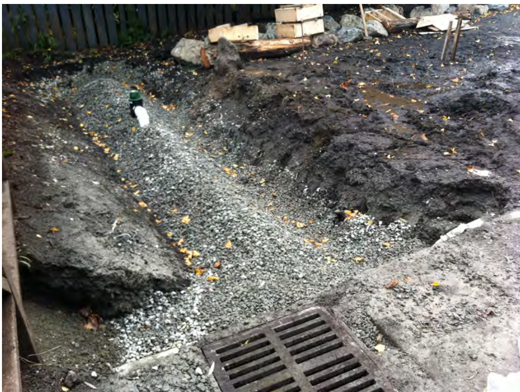
Figure 4.34: The under drain and overflow drain completed
