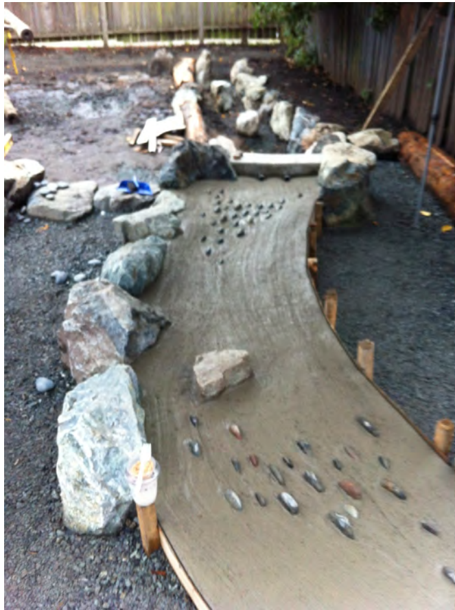
Figure 4.32: Concrete with embedded stones and the bioswale behind
