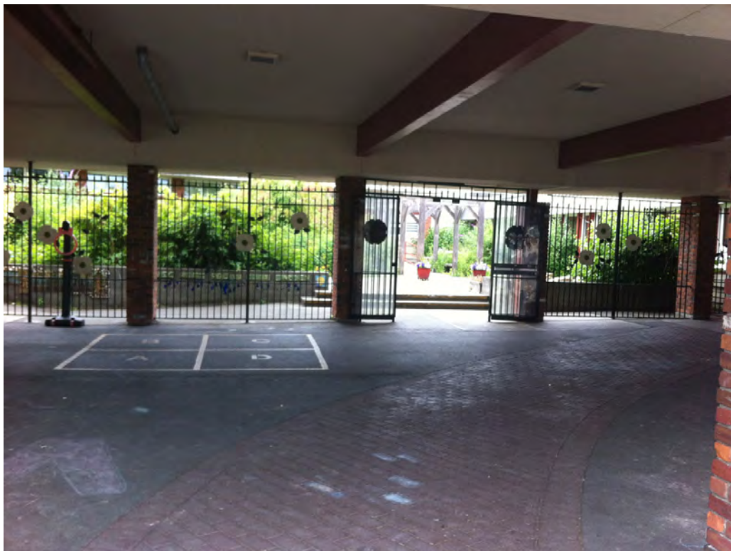
① Figure 3.30: Decorative metal fence enclosing the garden
