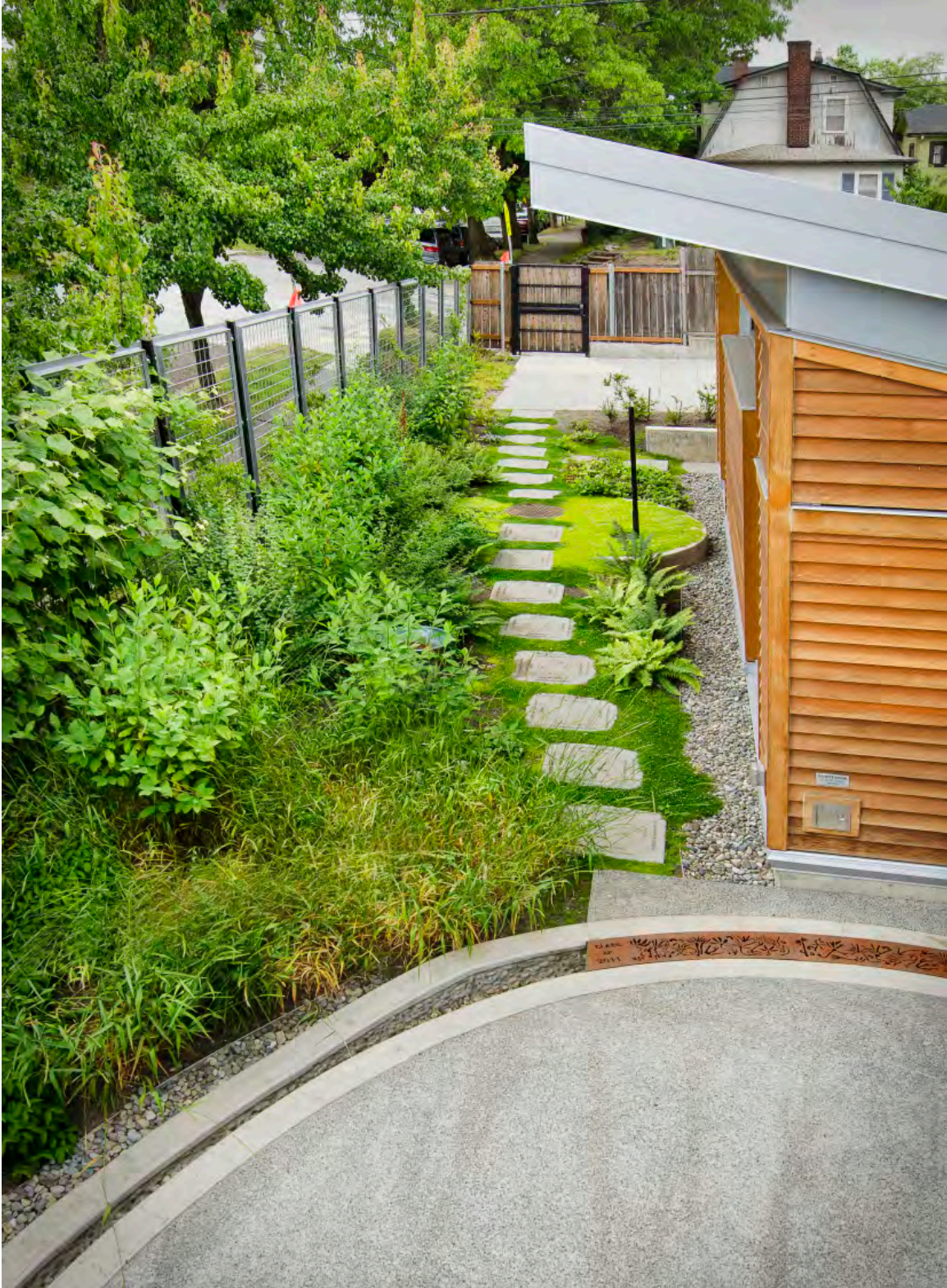
⑥ Figure 3.11: The rain garden, ethnobotanical garden and the below ground outdoor cistern with water level measurement stick (GGLO, 2013b)
