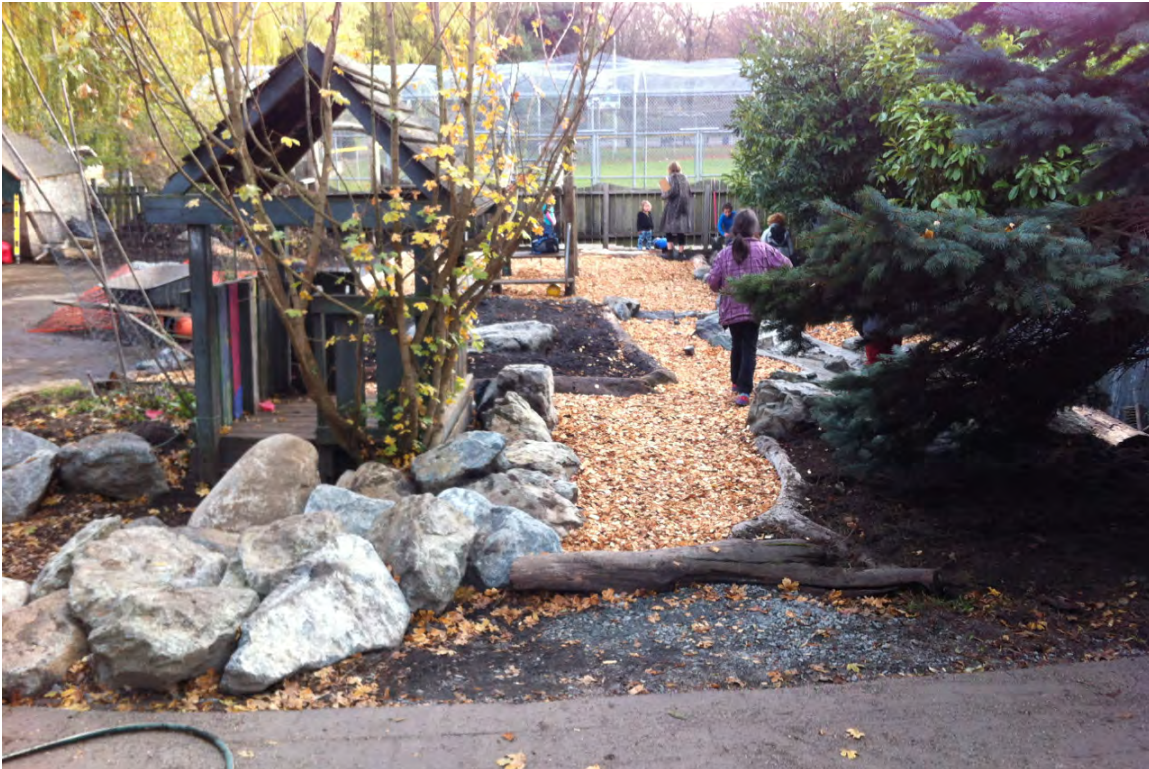
Figure 4.51: A number of extra boulders were used in this area and woodchips were placed throughout the play area.
