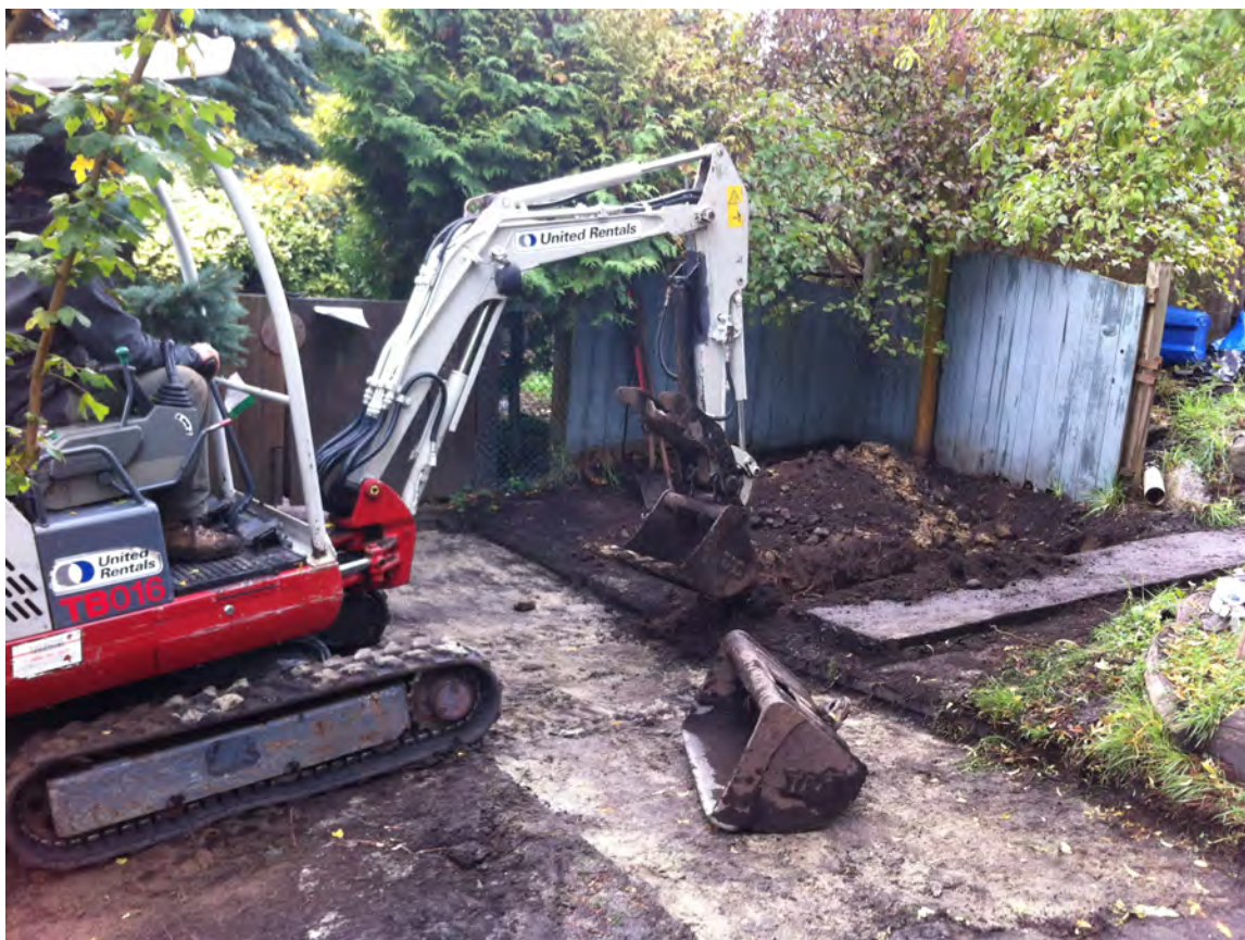
Figure 4.28: Excavating the trench for the underground pipes
