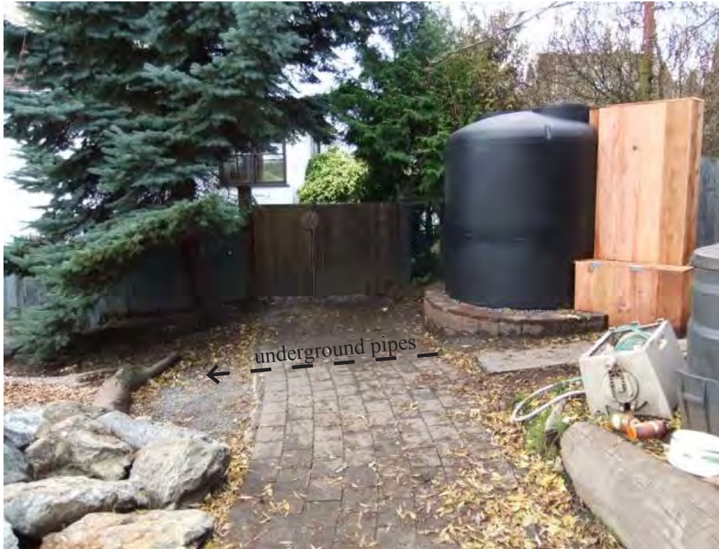
Figure 4.42: The cistern with protective wooden enclosure around the pipes, repaved pathway with improved grading and underground pipes.
