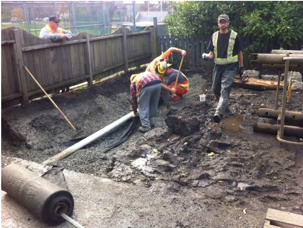
Figure 4.33: The City of Victoria installing the drainage for the rain garden
