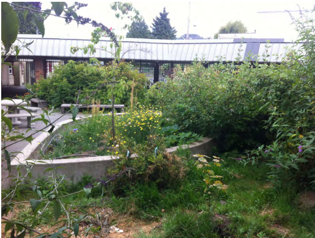
⑥ Figure 3.35: Rain garden enclosed in concrete wall
