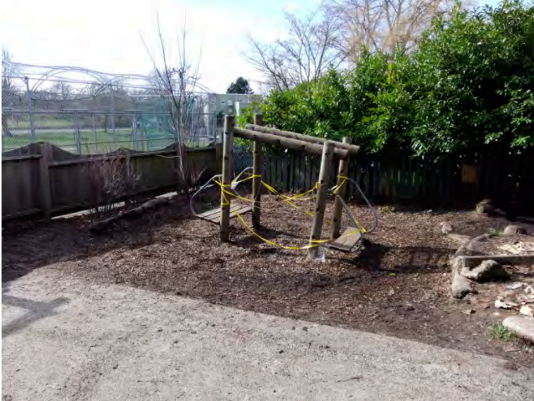
Figure 4.6: Site photo 3.1: Sinking monkey bars and water logged lower play area
