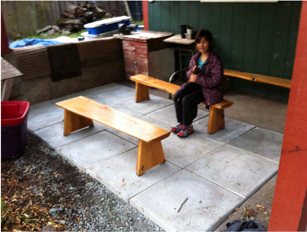
Figure 4.49: Pavers under deck
