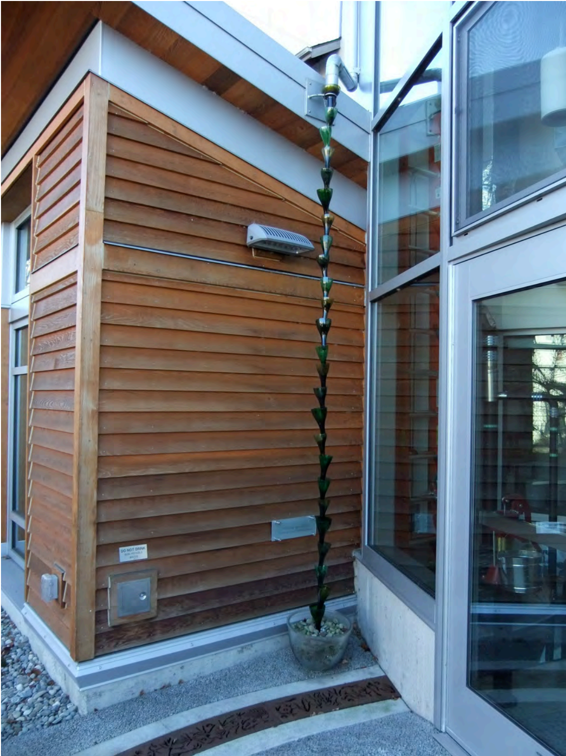
5 Figure 3.10: A decorative wine-bottle rain chain drains a section of the roof into the outdoor runnel
