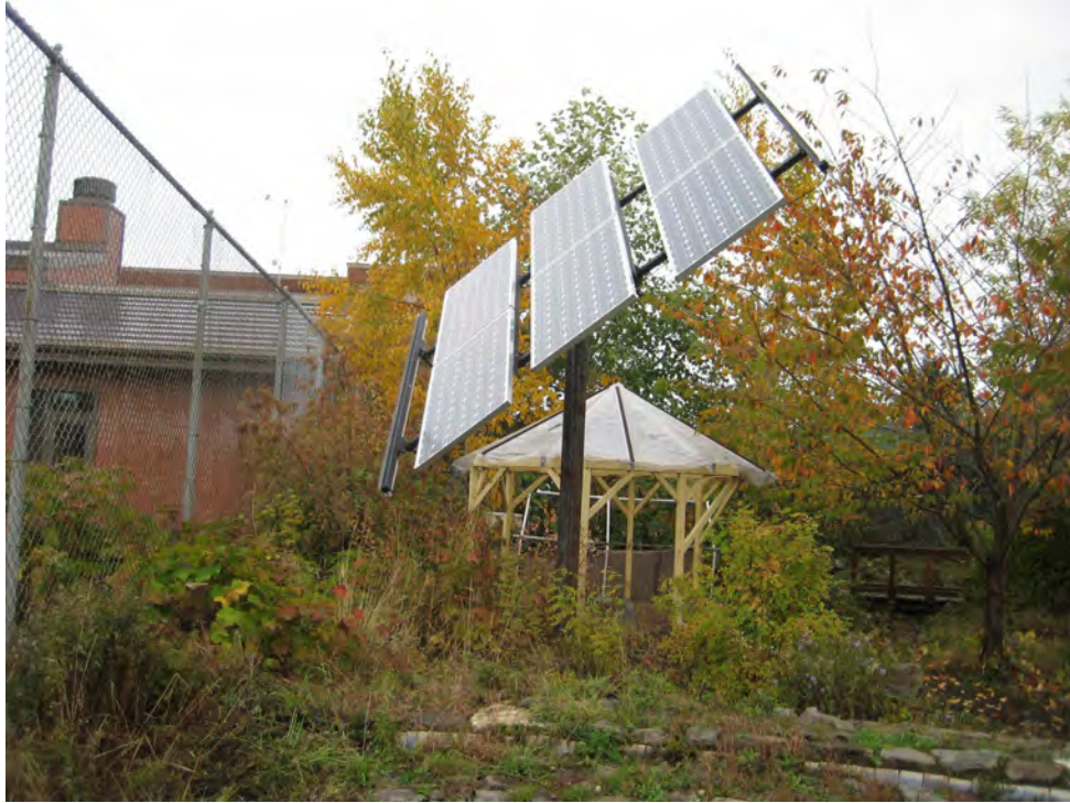
3 Figure 3.20: Solar panels, donated by Portland Electric, pump water through the flowform to aerate the water in the pond.
