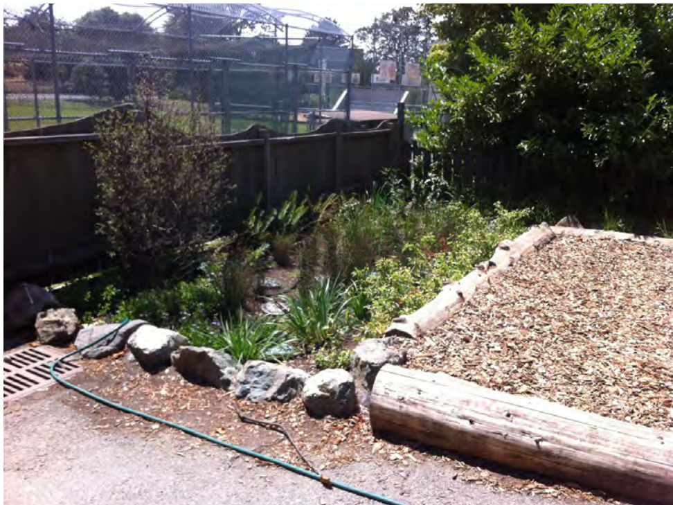
Figure 4.47: The rain garden, July 2015
