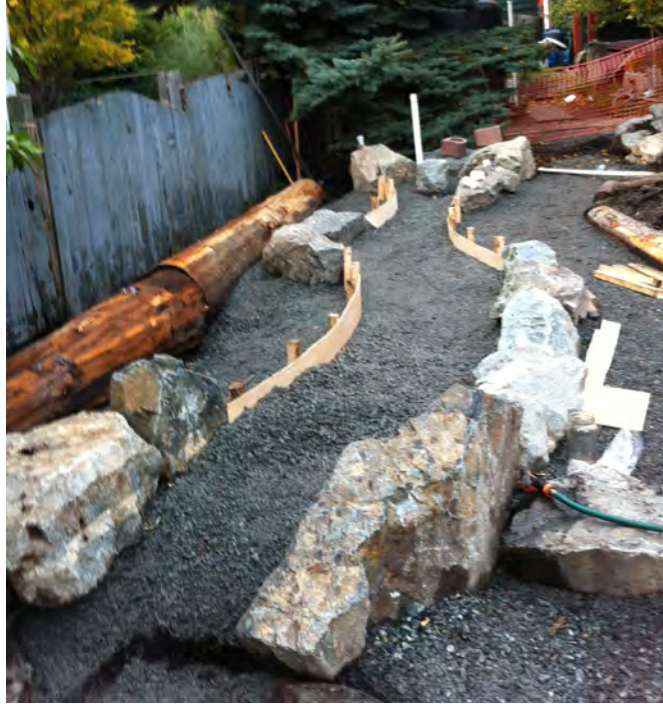
Figure 4.31: The base work for the concrete play-swale
