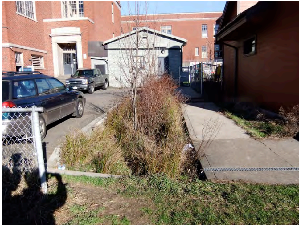
① Figure 3.18: Water from the parking lot collects into a bioswale which overflows into the swale and to the wetland, bypassing the pond to keep out pollutants from cars.
