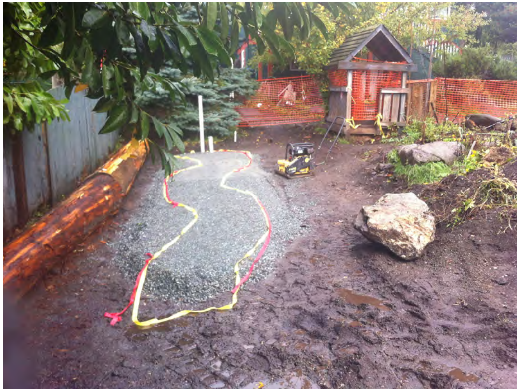
Figure 4.30: Laying out the play-swale.
