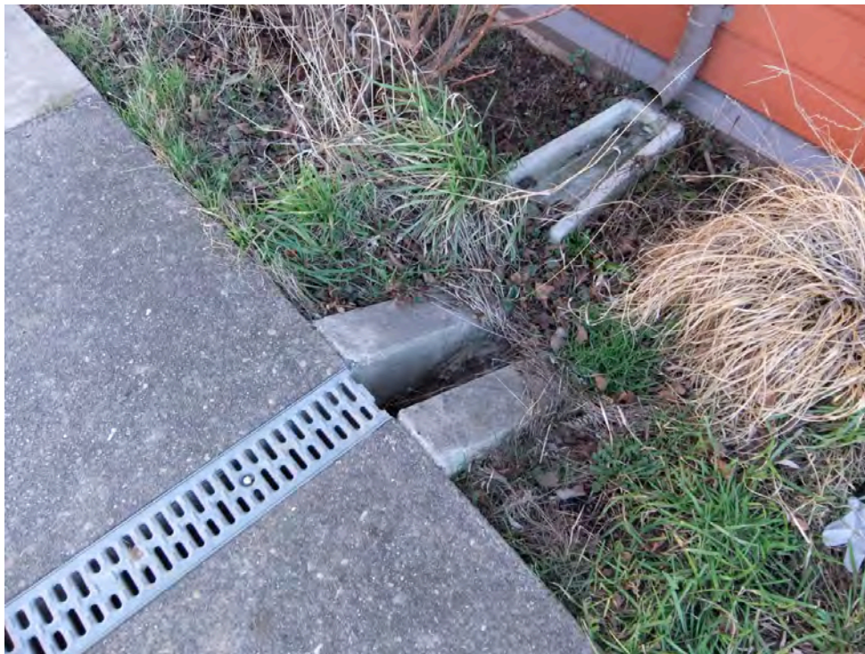
② Figure 3.19: Some of the water collected off the building adjacent to the water garden goes to the bioswale while most goes to the cisterns and the pond.
