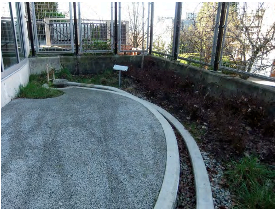
7 Figure 3.12: When both cisterns are full, water backs up into this runnel, pouring into the rain garden. This area of permeable concrete serves as an outdoor classroom.
