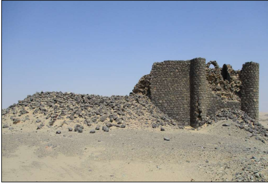
Pl 13. A. The external side of the southern wall of the fort.
