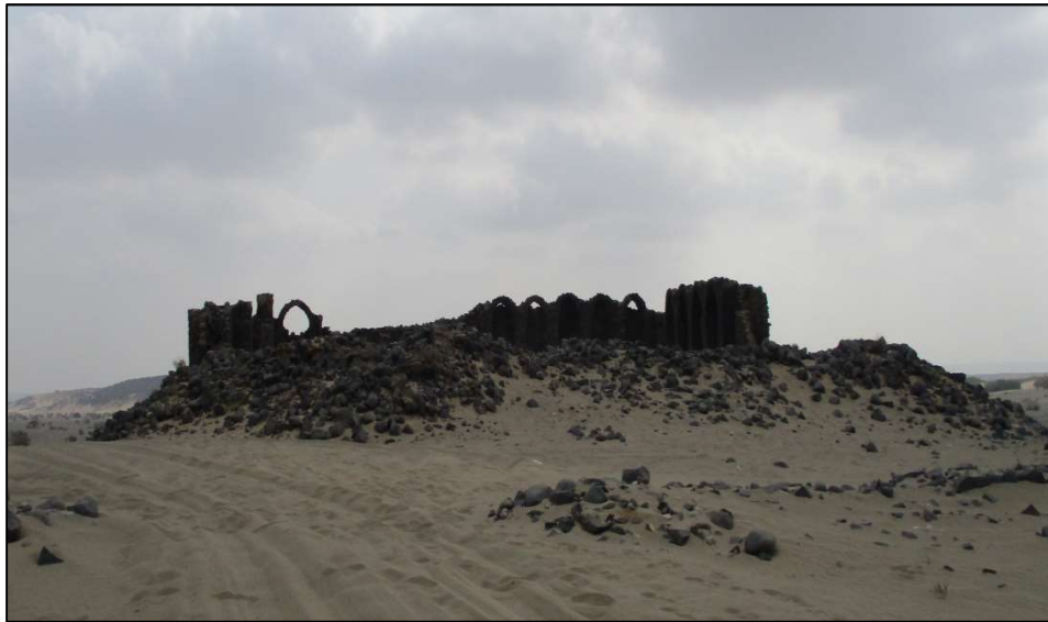
Pl 9. B. The external side of the western wall of the fort.
