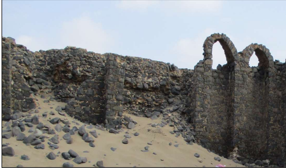
Pl 9. A. The interior side of the northern wall of the fort.
