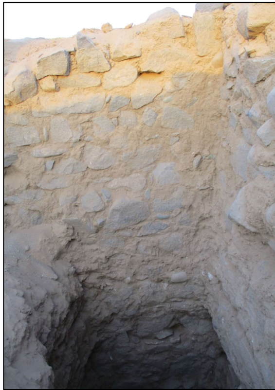
P1 20. B. The wall height of the architectural unit after the excavation is completed.
