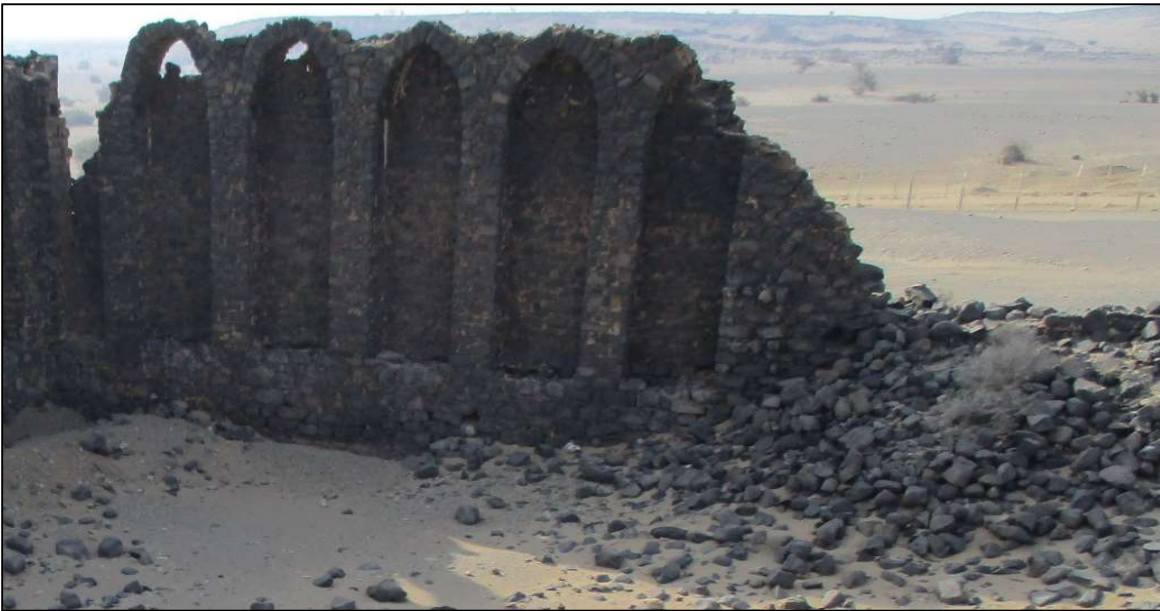
Pl 13. B. The interior side of the southern wall of the fort.
