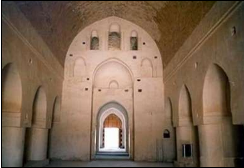
Pl 25. A. Abbasid pointed arches in Qasr al-Ukhaidir, 8 th century. (Shafi'i, Pl. 178).
