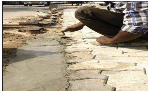
Figure 13: Mortar filling near edges
