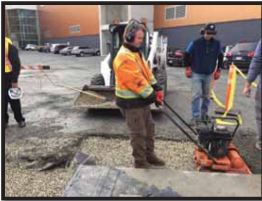
Figure7. Gravel Compaction
