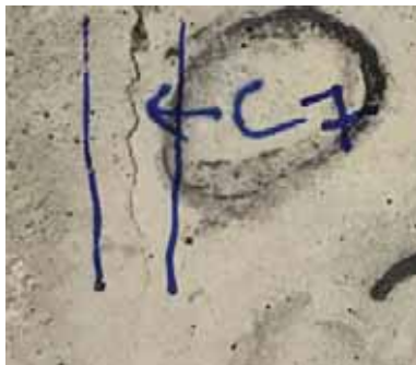
Fig 7: Induced Crack in a Cube
