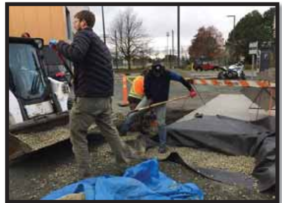
Figure6. Gravel Placement
