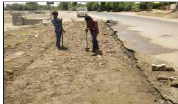
Figure 6: Levelling & Compaction of Earth using Tamper
