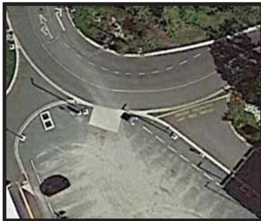
Figure3. Top view of site
