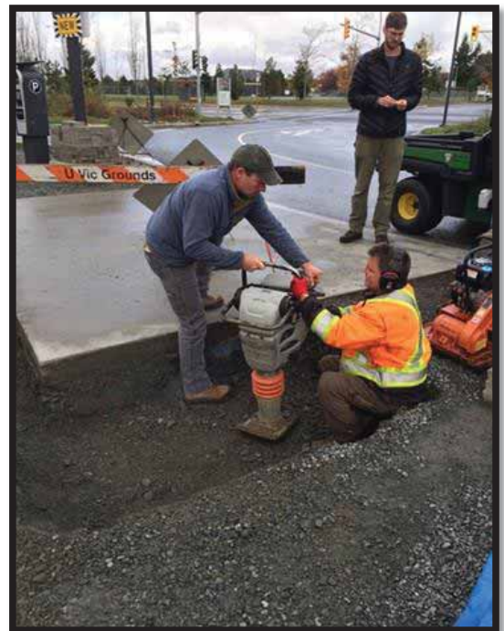
Figure5. Soil Compaction
