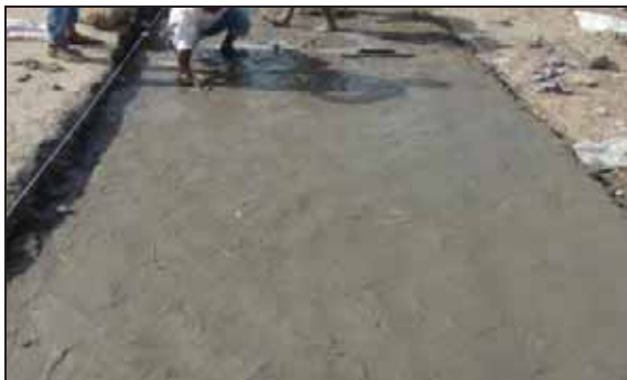
Figure 10: Laying of Portland cement concrete
