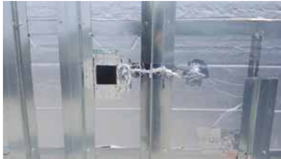
Figure 4. External Heat Flux, Temperature and Pressure Installation
