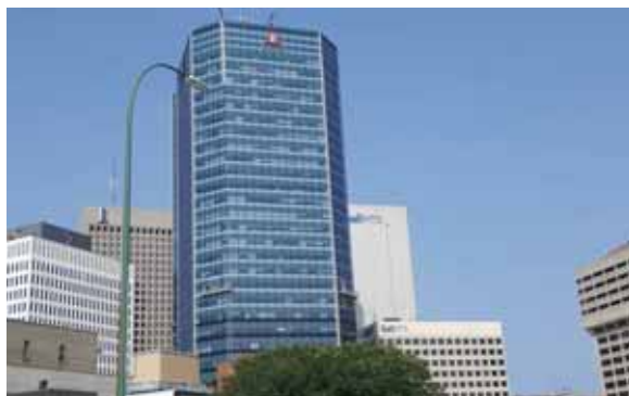
Figure 5. 32-Storey High-Rise Building
