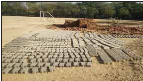
Figure 4: Casting of alkali activated concrete paver blocks
