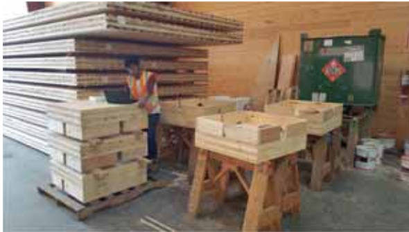
Figure 5. Six Additional Off-cuts Instrumented on May 27th, 2016
