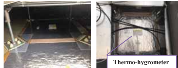
Fig6: Construction in real environment of VIP
