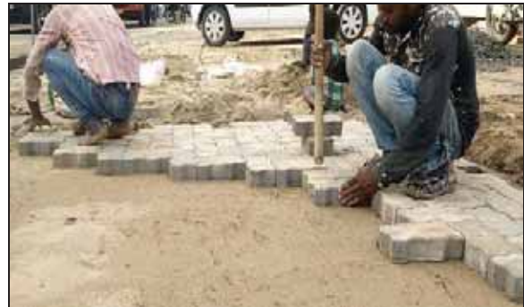
Figure 12: Laying of pavers in herringbone pattern
