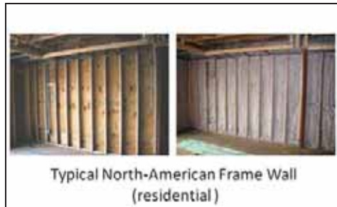
Figure 2. Frame walls
