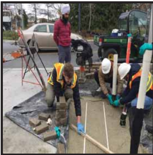
Figure8. Bedding Soil Placement
