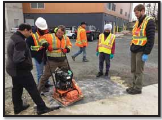
Figure 10. Final Compaction
