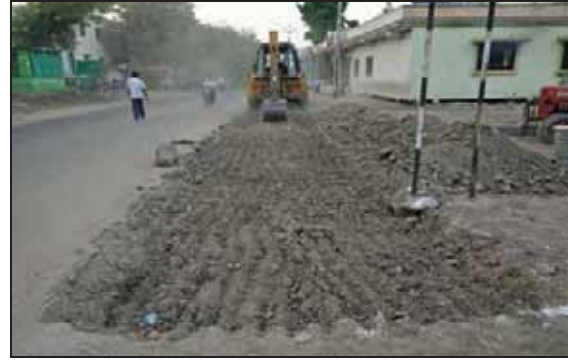
Figure 5:Excavation of 200 mm depth using backhoe
