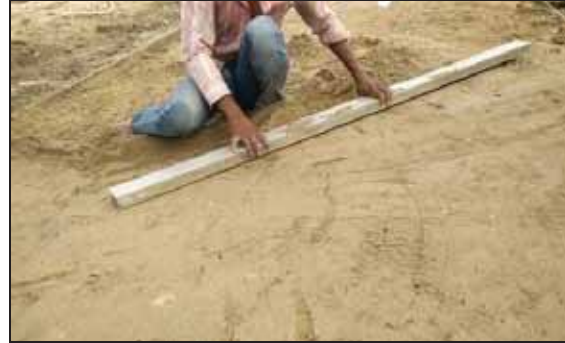
Figure 11: Laying of 40 mm Sand Bedding & Levelling
