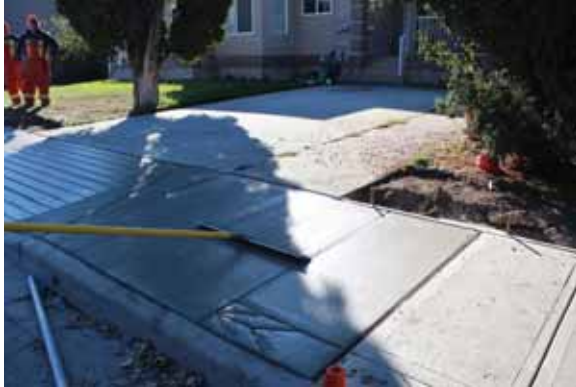
Fig 1: Construction of sidewalk with RC
