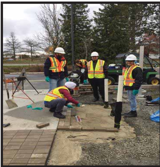
Figure9. Paver block placement
