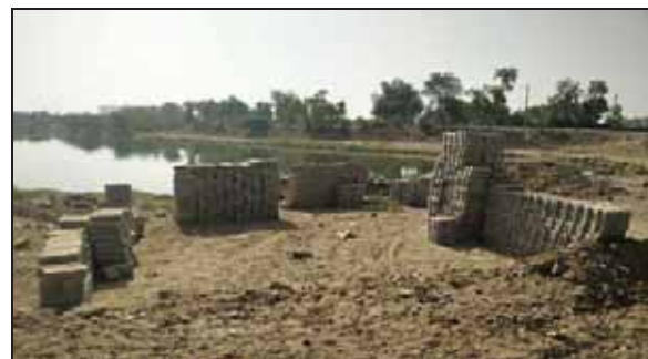
Figure 7: Storage of paver blocks
