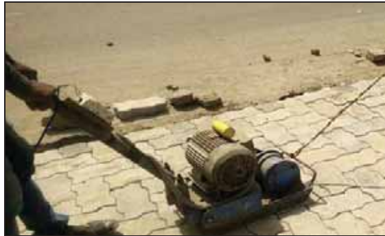
Figure 14: Compaction on paver blocks
