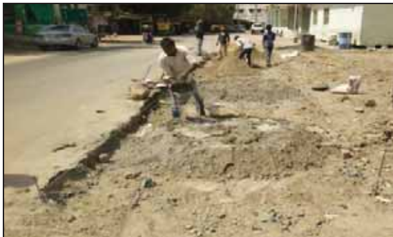
Figure 9: Preparation of M10 grade concrete
