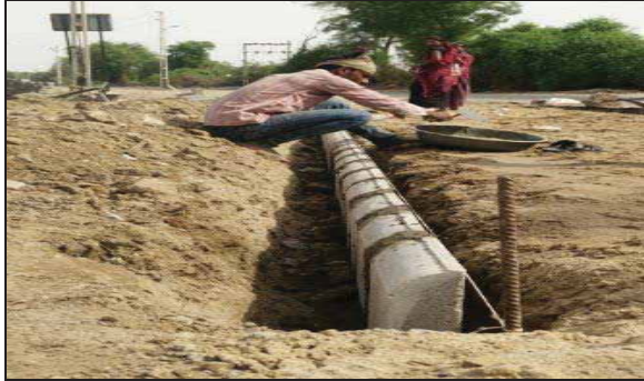
Figure 8: Laying of 12 inch kerb stones
