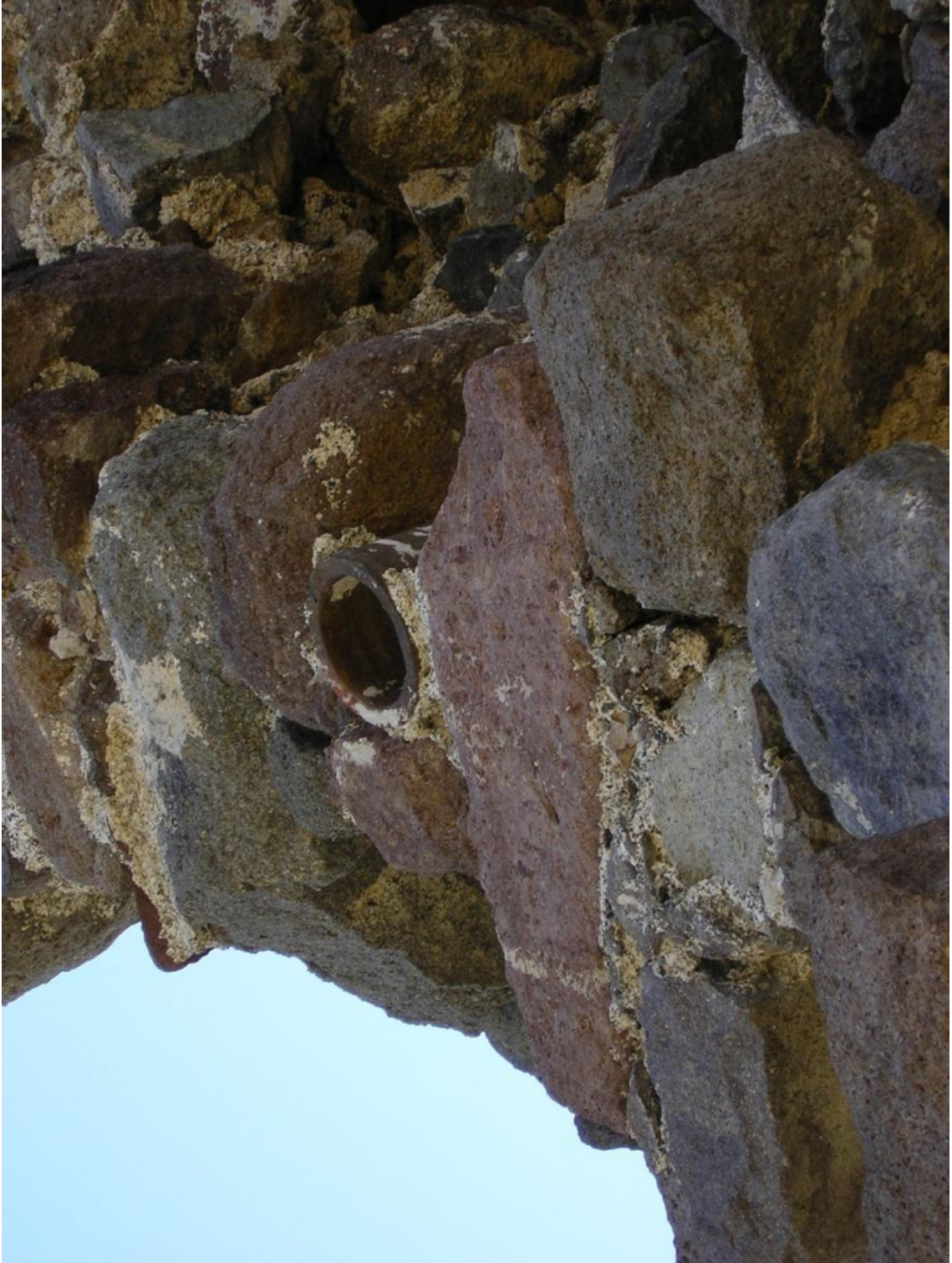
Figure 7.5: View of Terracotta Pipe in situ in WNW-Side of Tower
