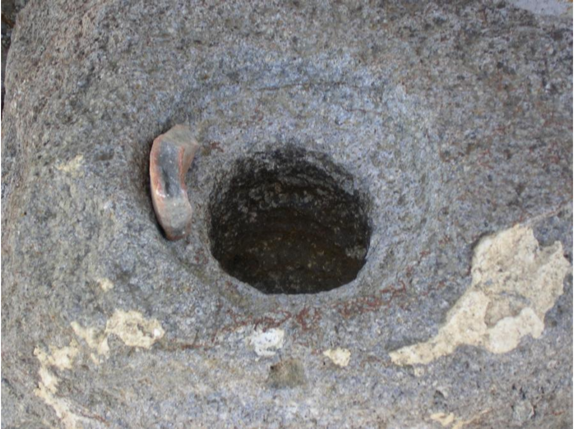
Figure 16.1: Pipe Hole at Methymna
