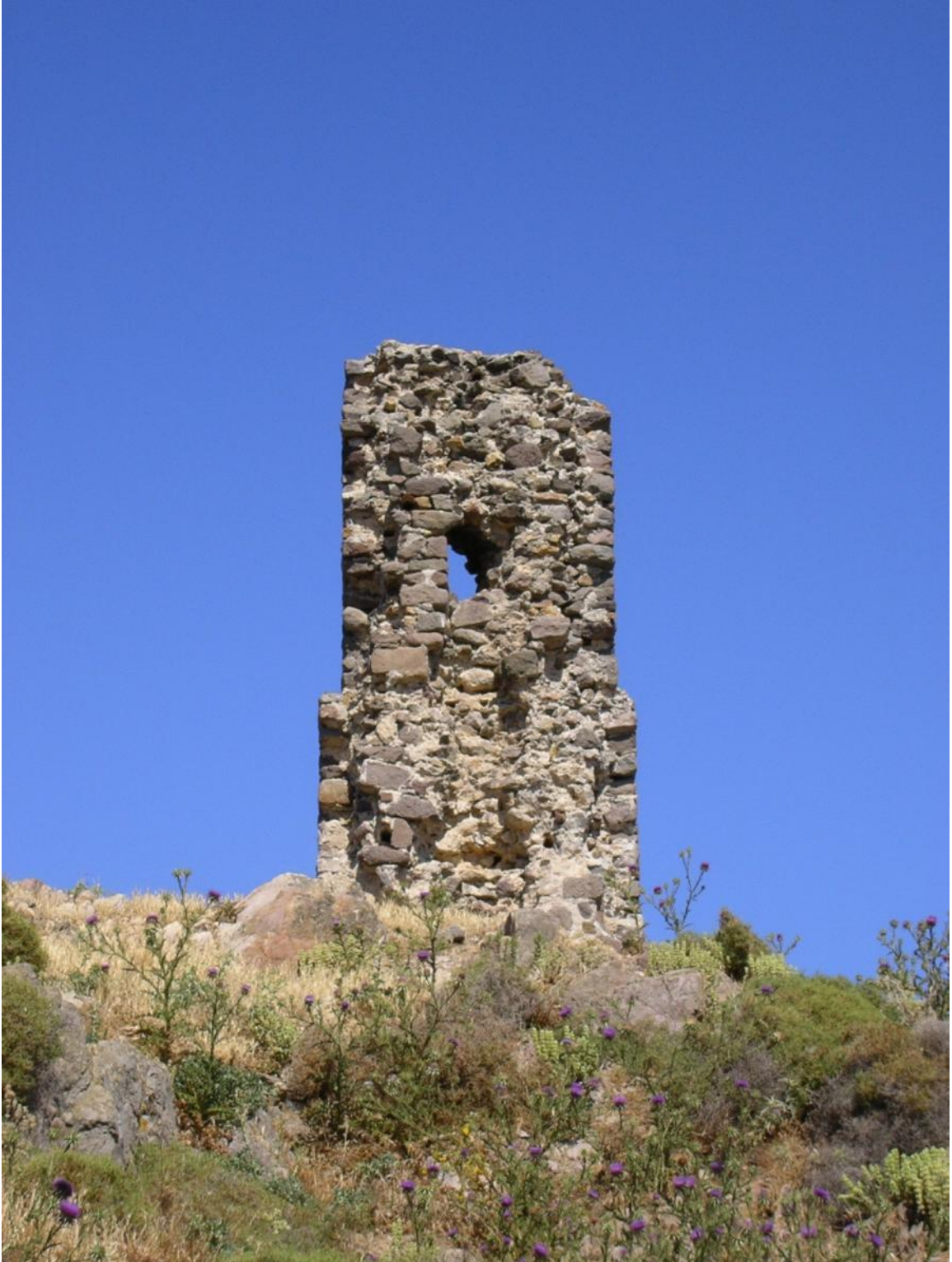
Figure 7.3: View of Tower from ESE
