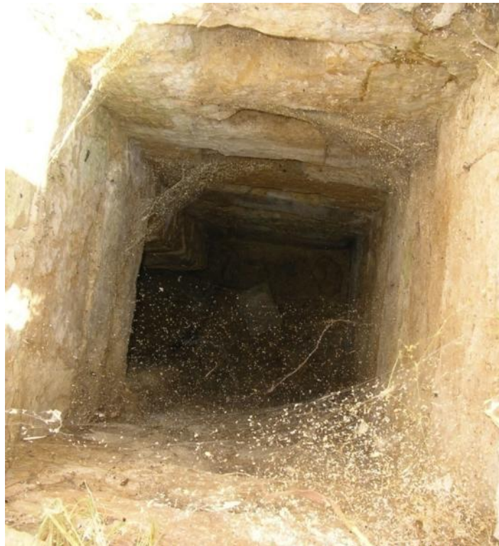
Figure 10.4: Interior of the only unsealed manhole
