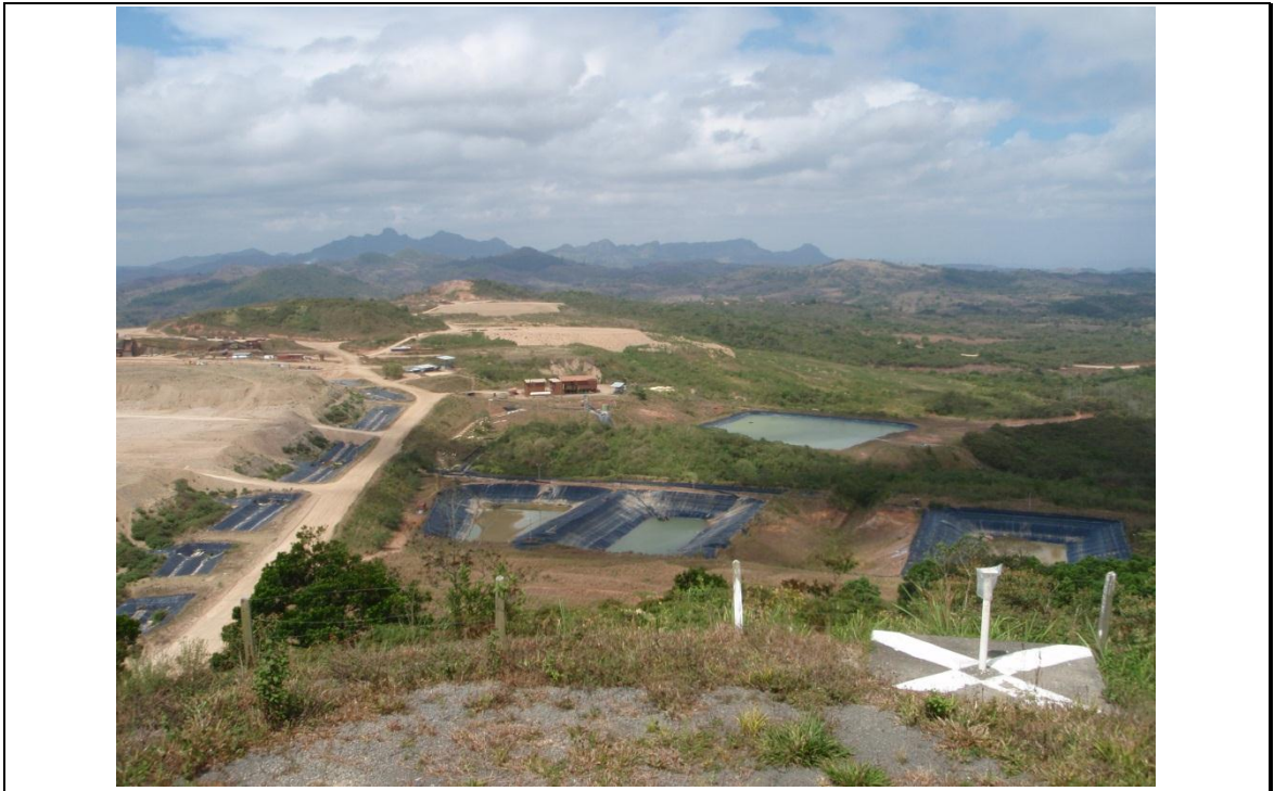
Figure 2-6. La Libertad Mine
