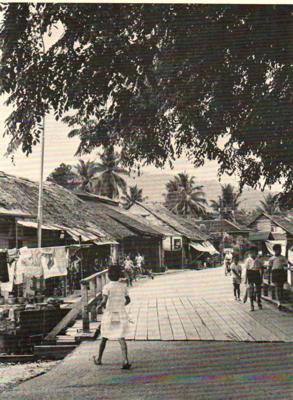
New Village entrance
