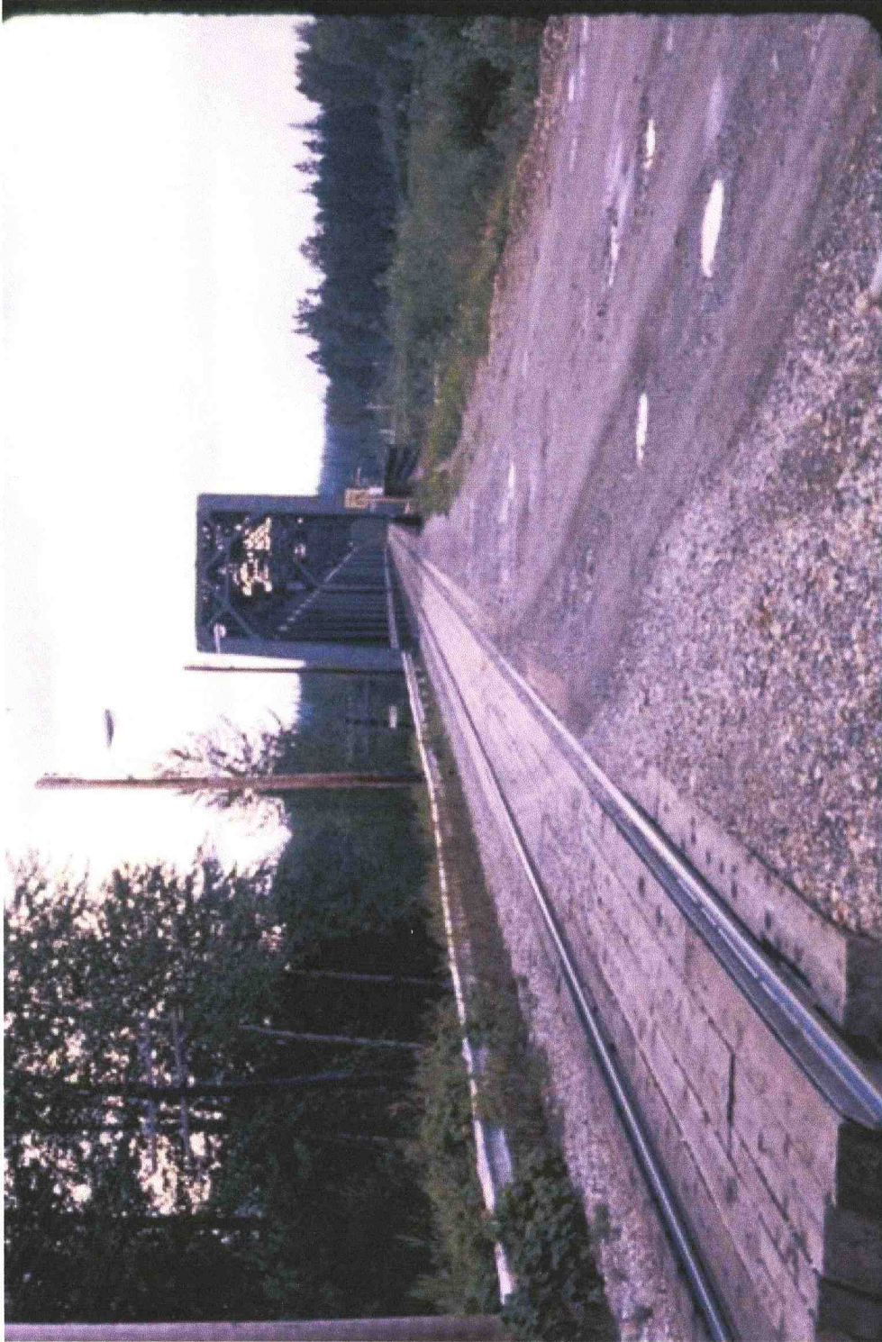
IMAGE 20 Looking west over the dual-use bridge that carries both the Upper Fraser road and the Canadian National Railways line across the Fraser River at Hansard, 1976. Photograph by Kent Sedgwick. Courtesy of Kent Sedgwick and UNBC's Upper Fraser Mill Town Historical Geography Project.
