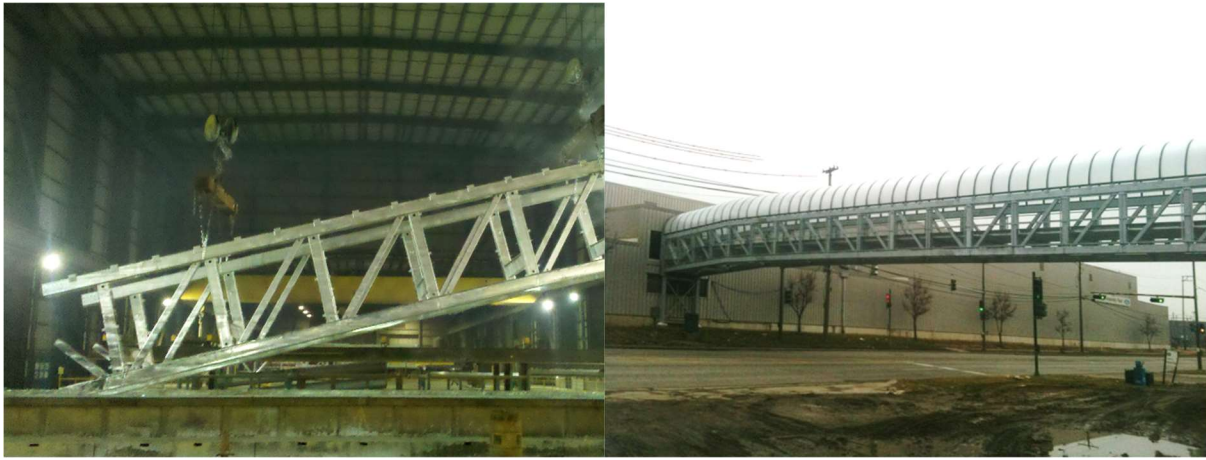
Fig. 1. Galvanizing of rectangular hollow section truss (Ford Pedestrian Bridge in Chicago, IL, United States) [Photo courtesy of American Galvanizers Association]
