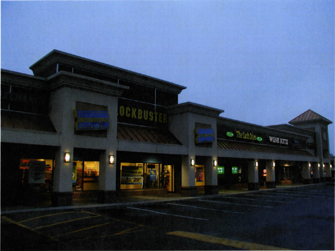
Figure 4.13 Terminal Park Mall, Island Highway, Nanaimo
