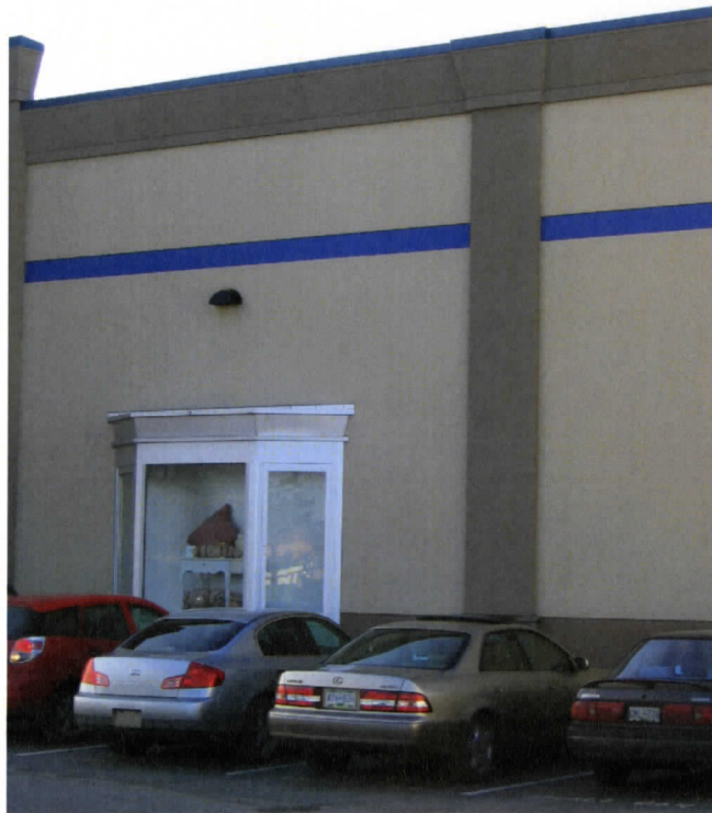
Figure 4.64 Detail, Façade, Home Outfitters, Millstream Road, Langford.
