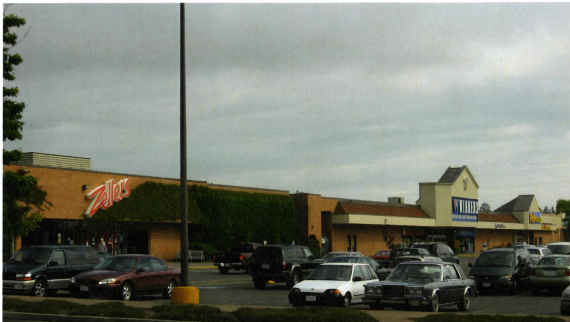
Figure 4.17 Upper Level Façade, Tillicum Mall, Saanich.
