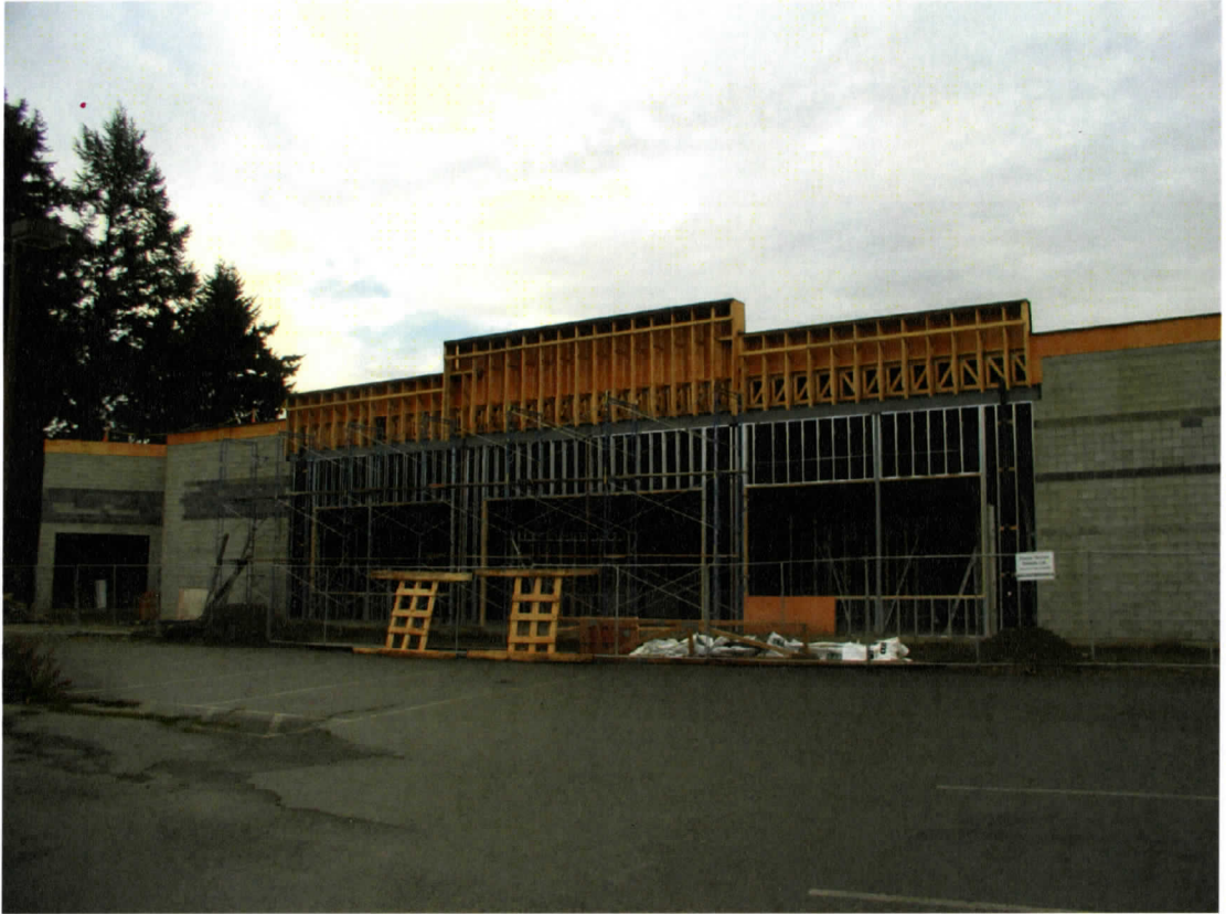
Figure 4.23 Facade, The Brick, Frontage Road, Duncan.
