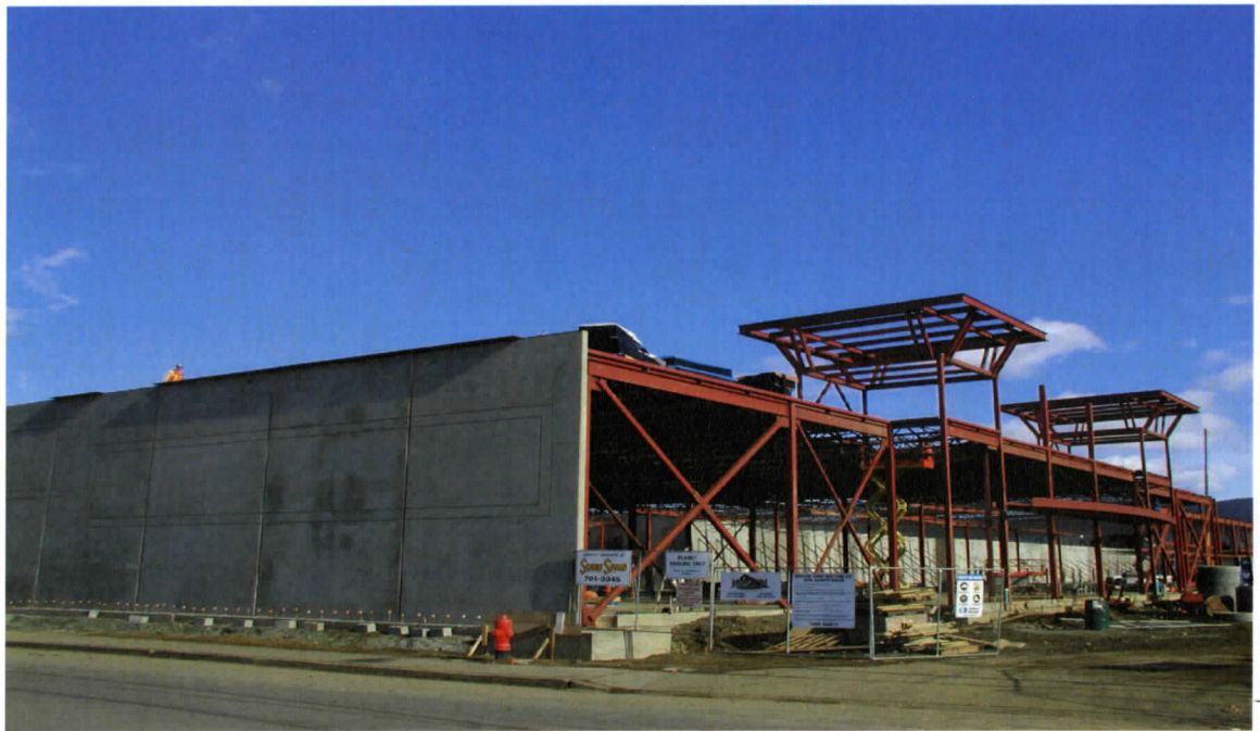
Figure 5.3 Power Centre Construction, Village Green Mall, Highway One, Duncan.
