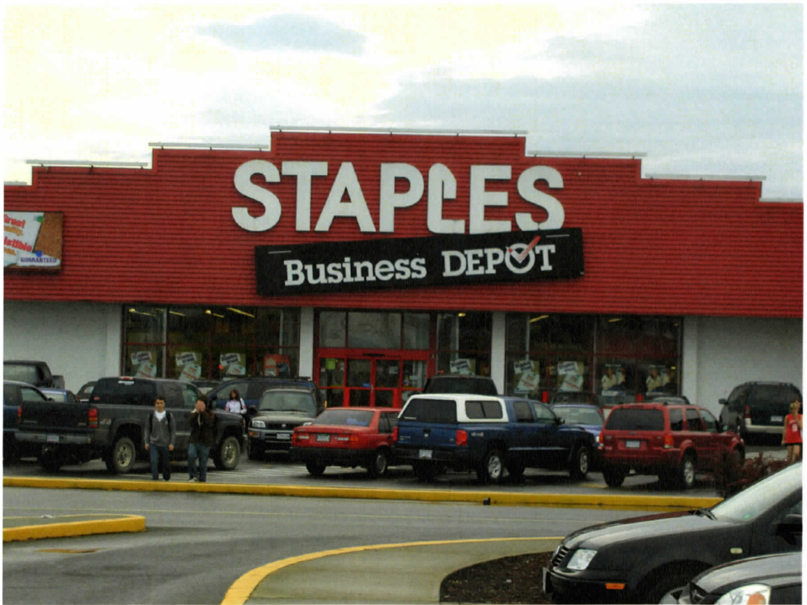
Figure 4.28 Crow Step False Front, Staples, Duncan Mall, Duncan.
