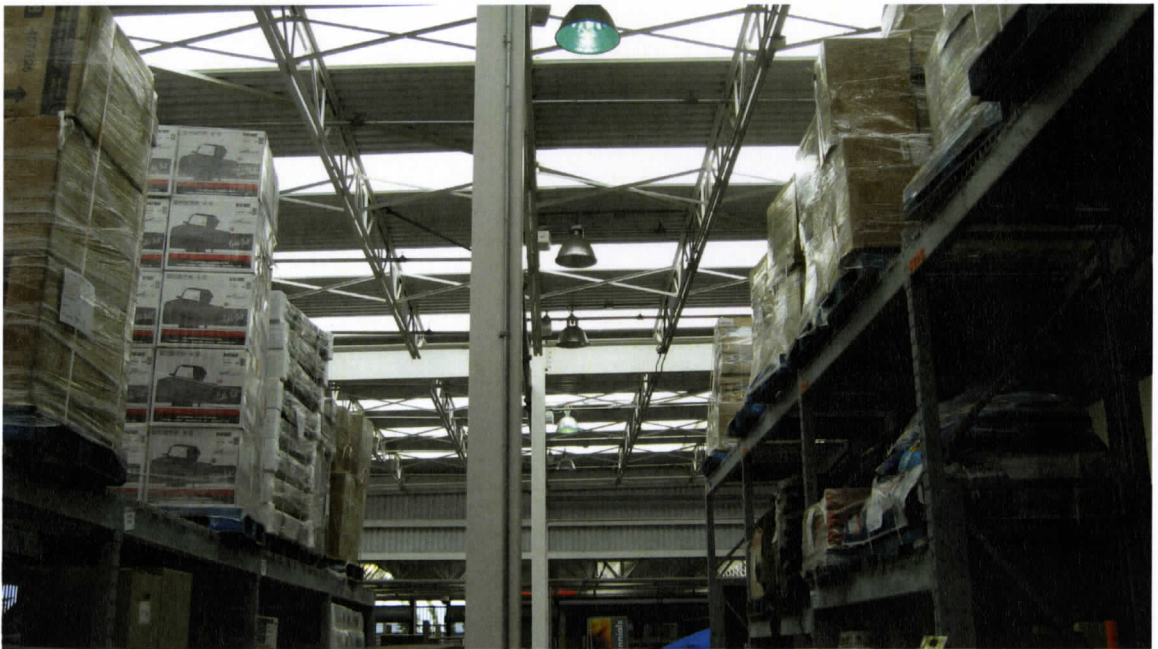
Figure 4.34 Steel Frame, Garden Centre, Home Depot, University Heights Shopping Centre, Saanich.
