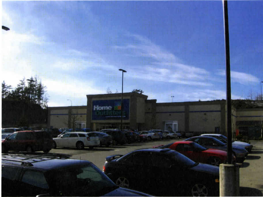
Figure 4.63 Façade, Home Outfitters, Millstream Road, Langford.
