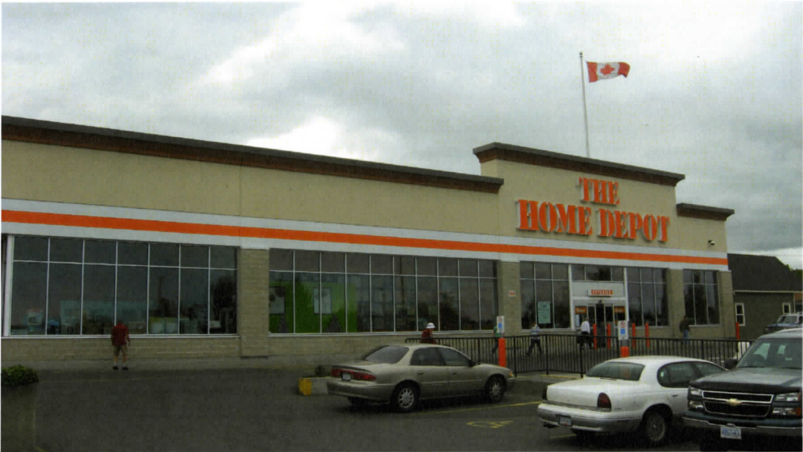
Figure 4.36 Façade, Home Depot, University Heights Shopping Centre, Saanich.
