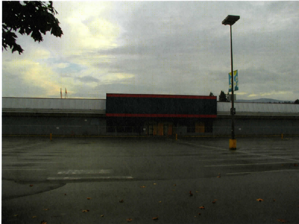
Figure 4.3 Former Wal-Mart, Duncan Mall, Duncan.
