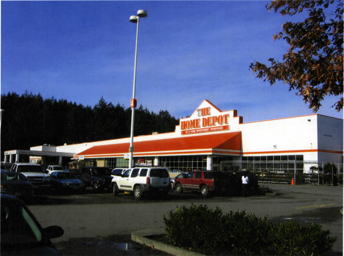
Figure 4.37 Façade, Home Depot, Millstream Road, Langford.
