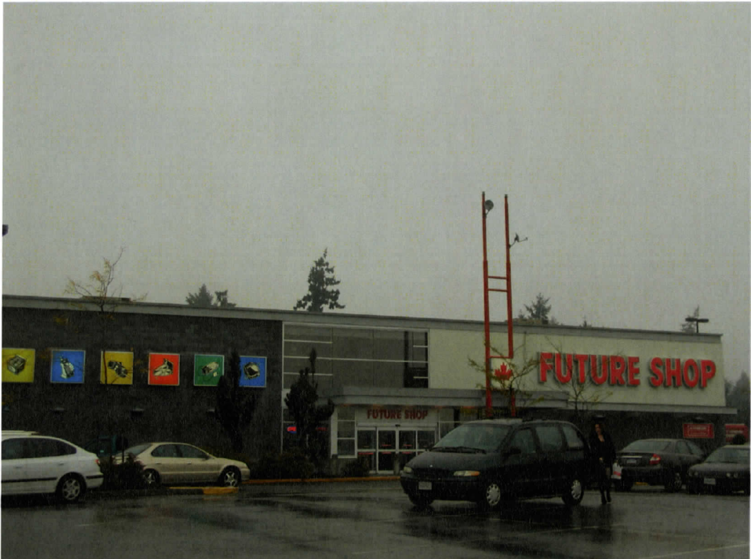
Figure 4.62 Façade, Future Shop, Country Club Centre, Island Highway, Nanaimo.
