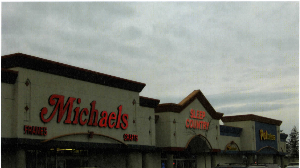
Figure 4.72 False Fronts, Mary Ellen Crossing, Island Highway North, Nanaimo
