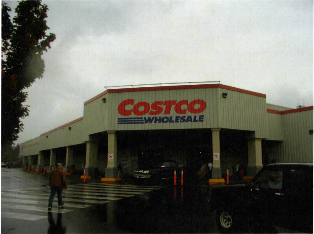
Figure 4.44 Entrance, Costco, Island Highway North, Nanaimo.
