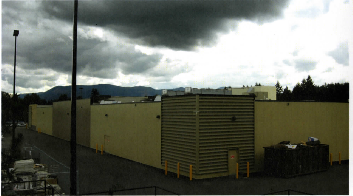
Figure 4.55 East Wall, Wal-Mart, Drinkwater Road, North Cowichan
