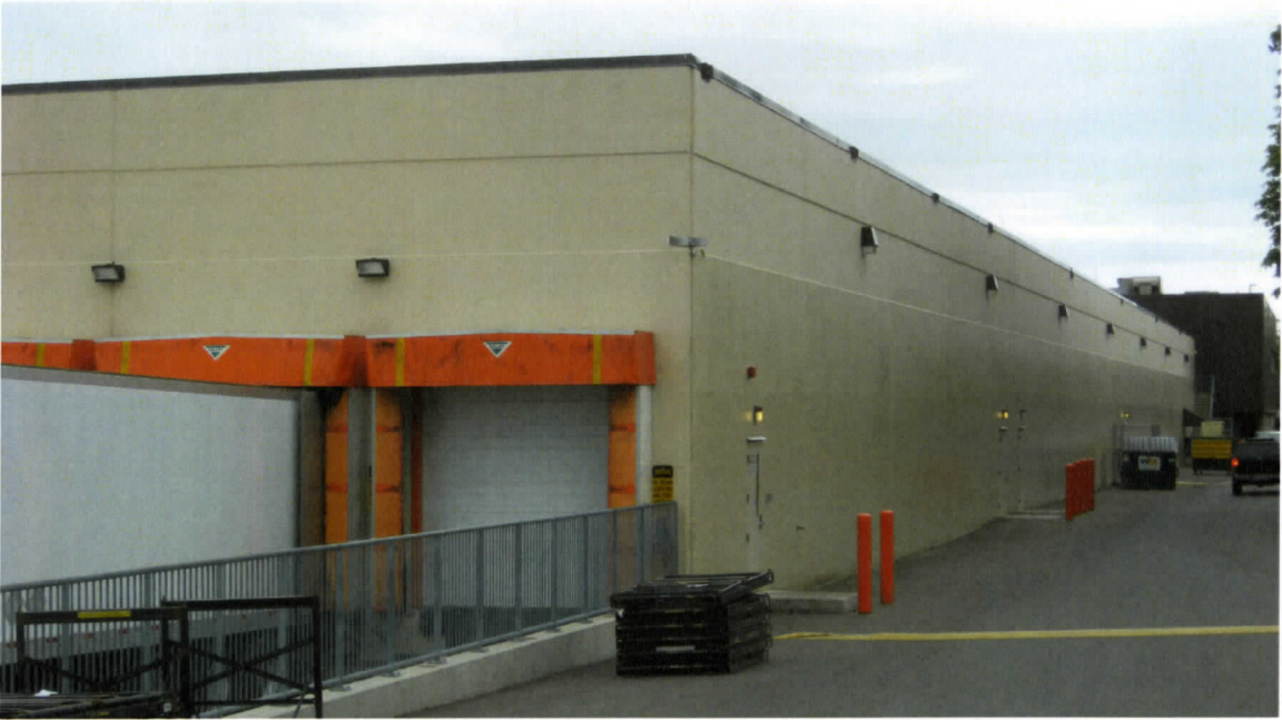
Figure 4.32 West Wall, Home Depot, University Heights Shopping Centre, Saanich.
