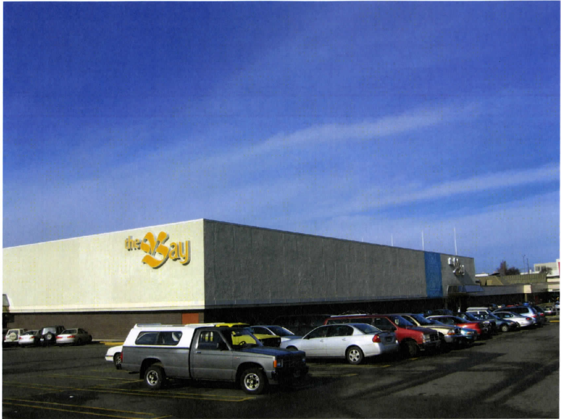
Figure 4.40 Hudson's Bay Company Store, Mayfair Shopping Centre, Victoria.
