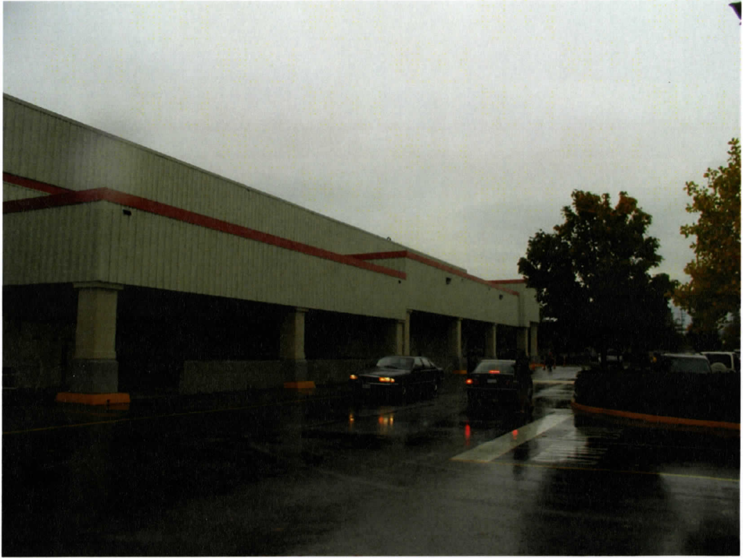
Figure 4.48 West Curtain Wall, Costco, Island Highway North, Nanaimo.
