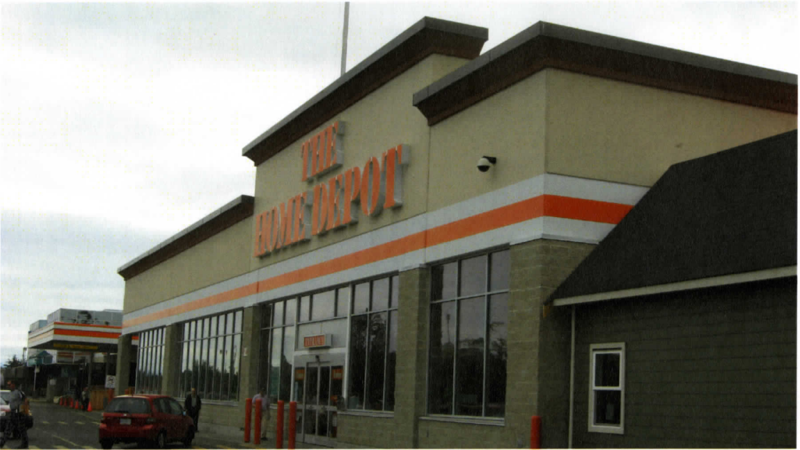
Figure 4.39 Façade, Home Depot, University Heights Shopping Centre, Saanich.
