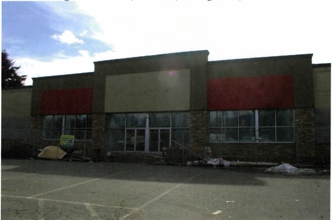
Figure 4.24 Detail, Facade, The Brick, Frontage Road, Duncan.
