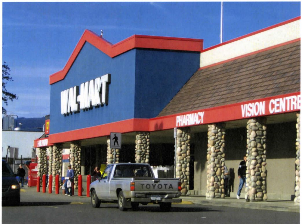
Figure 4.52 Façade, Wal-Mart, Attree Avenue, Langford
