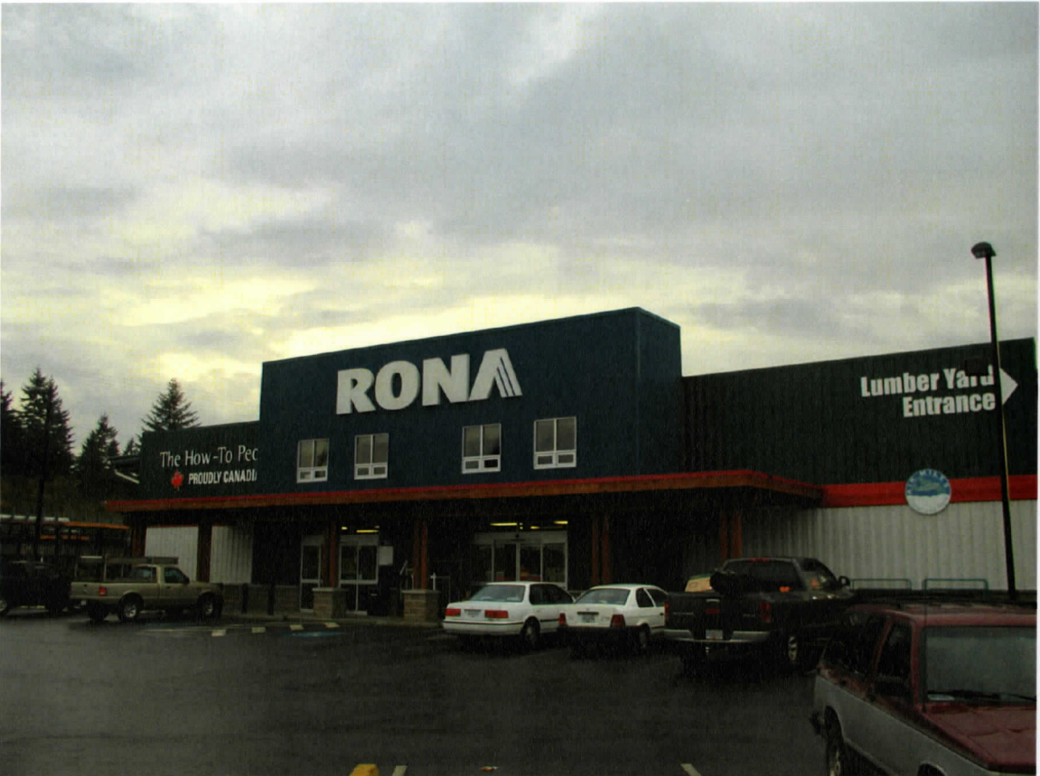
Figure 4.58 Rona Specialty Outlet, Island Highway, Cobble Hill.
