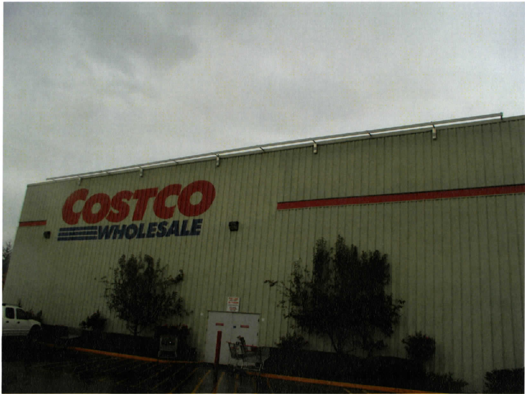
Figure 4.47 West Curtain Wall, Costco, Island Highway North, Nanaimo.
