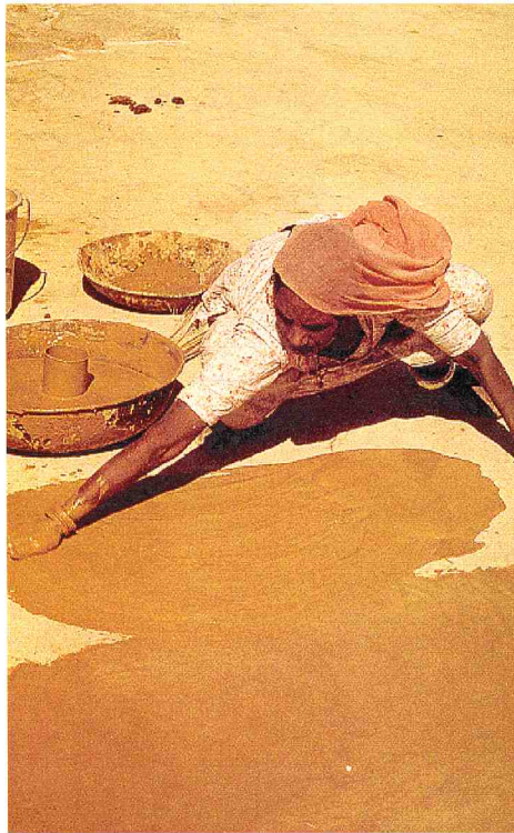
Figure 34 Preparing ground with mud dung mix for Mandana Rajasthan
