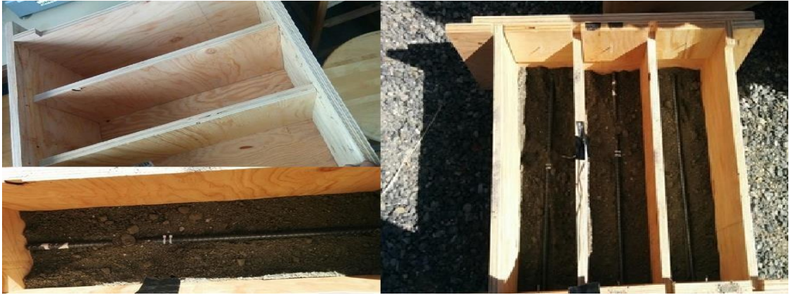
Figure 5 - Formwork of prisms including the rebar that is positioned
