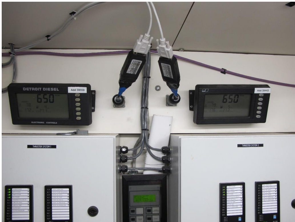
Figure A-3: Deutz 6 Pin Connections and HDV100A3 J1587/RS232 Converter
