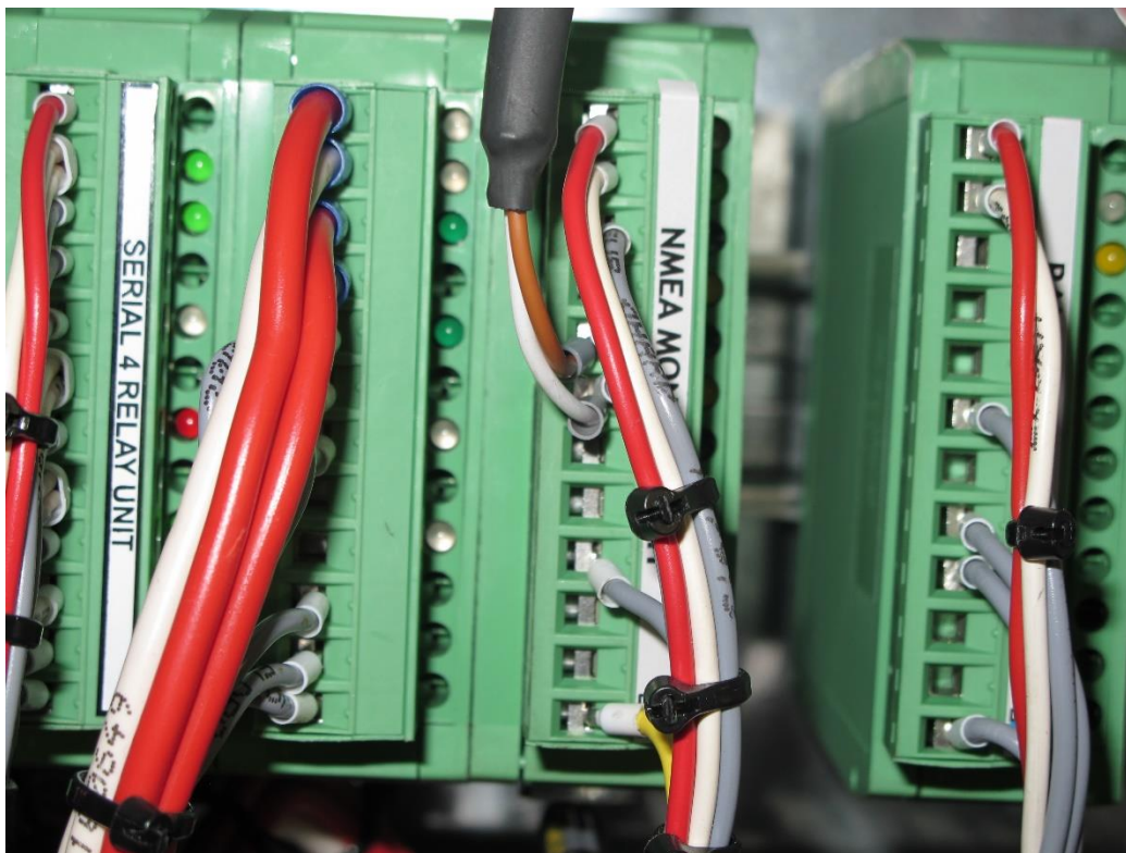
Figure A-7: Connection to HRP NMEA 183 Serial Bus
