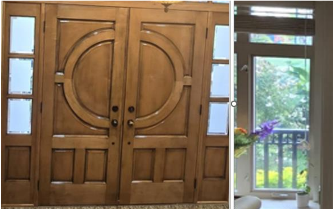
Figure 17: Door and Window (House-2)-No visible deficiencies
