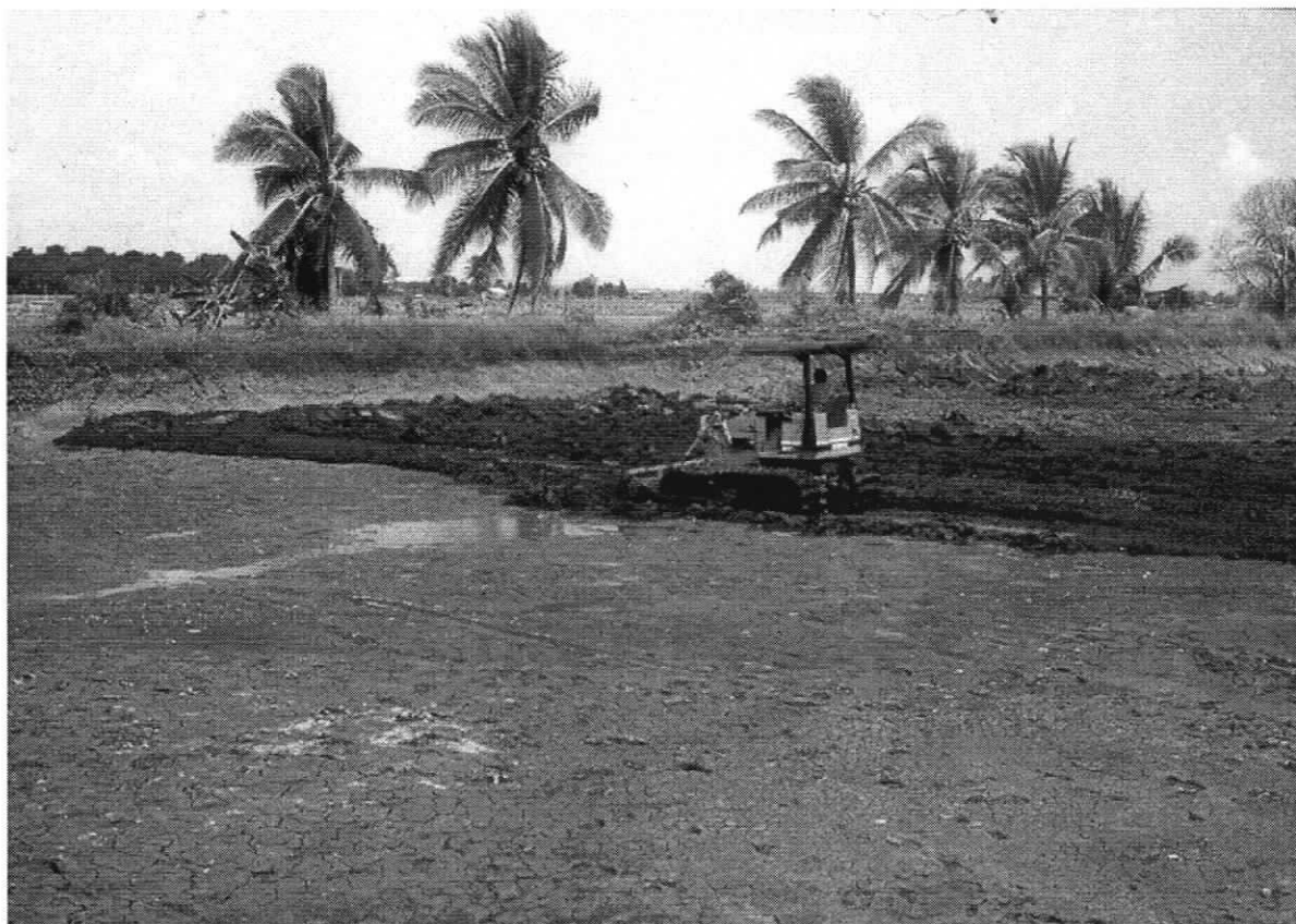
Figure 5.11 Sediment Removal from a Low-Salinity Shrimp Pond
