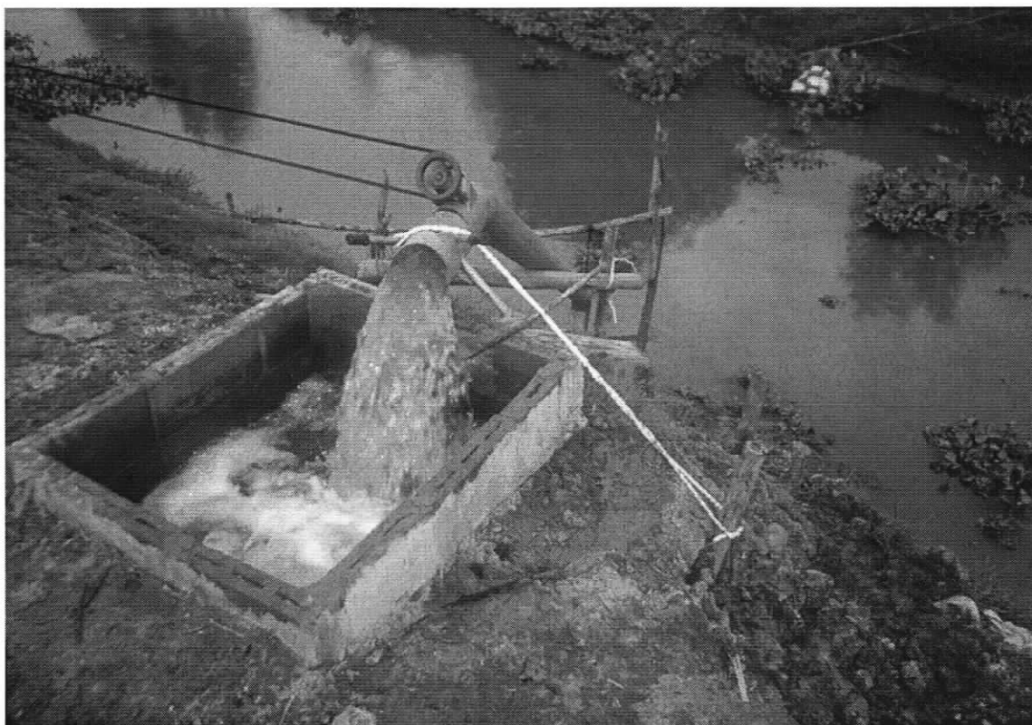
Figure 6.1 Freshwater Transfer from Small Irrigation Canal to Intake Structure for Low-Salinity Shrimp Farm
