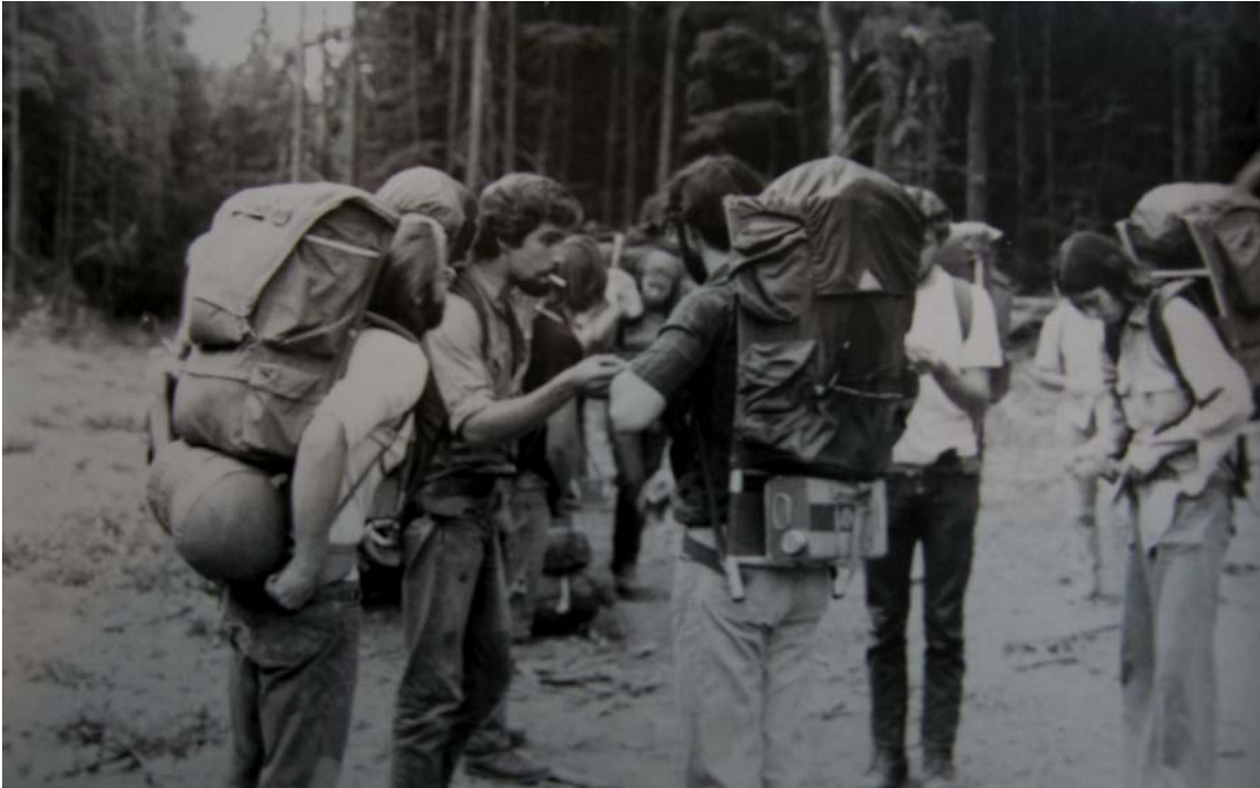
Picture 6.1: The Earl Grey Trail Building Crew.
