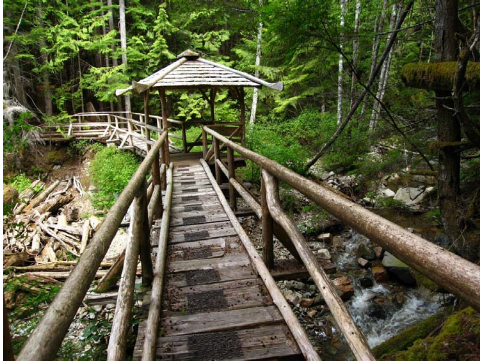
Picture 7.3: Edge's Way Bridge.
