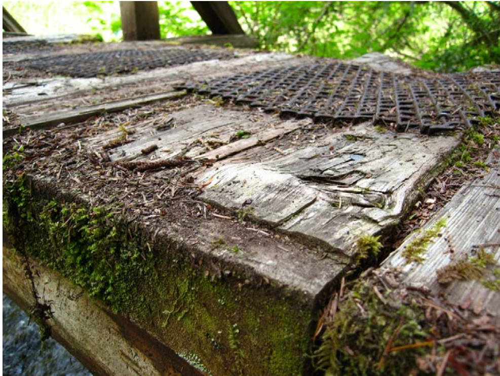
Picture 7.1: Decking on Squirrel Crossing Bridge. 47
