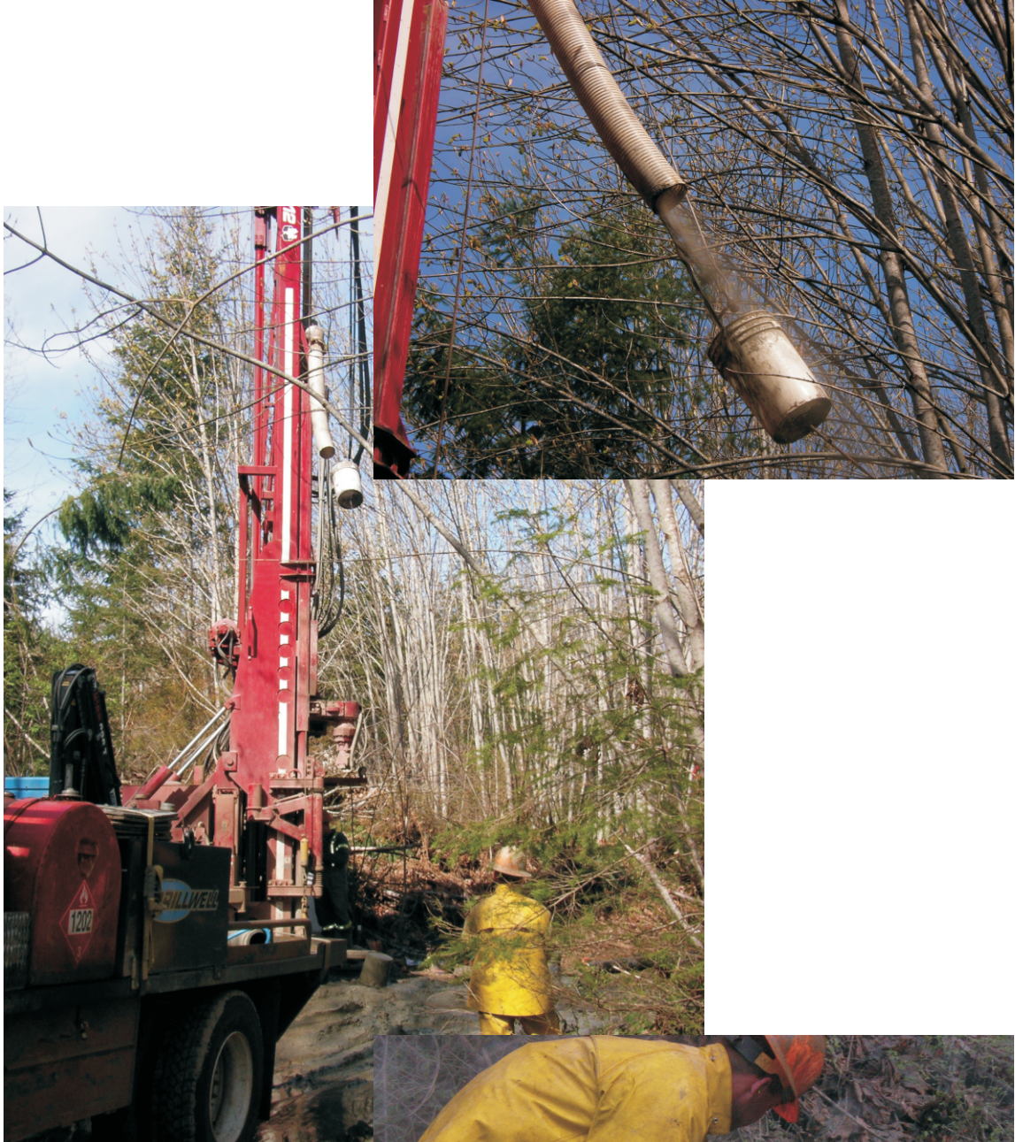
Figure 4.6. Drill cuttings sampling. These pictures are of a well drilled in Union Bay, southeast of Oyster River in the Comox Coalfield (UB-1, see Figure 2.8a in Chapter 2). The drilling and sampling procedure is the same for the Oyster River wells.
