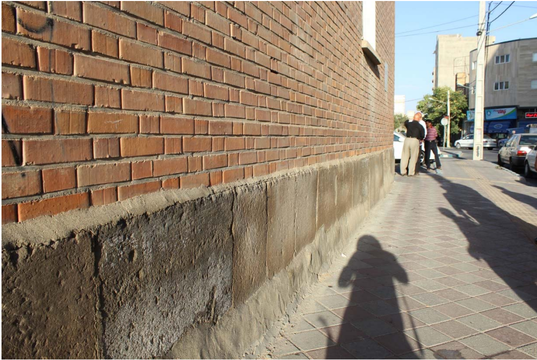
Figure 2-6: The grand mosque of al-Mahdiyya. The dark stones used in the lower parts of the walls seem to belong to an earlier building. Photo credit: Author.
