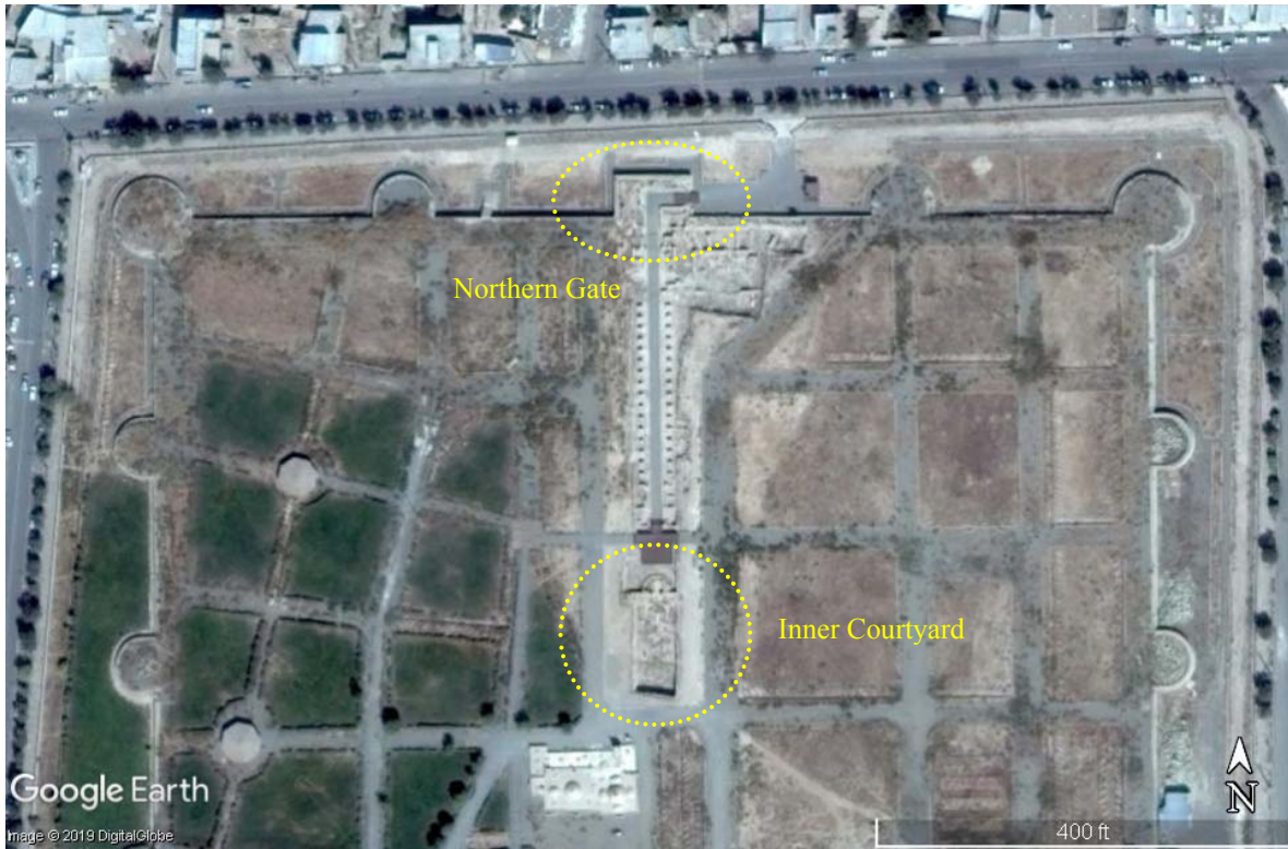
Figure 3-4: The northern gate, the passageway, and the inner courtyard. Photo credit: Google Earth. 2019 DigitalGlobe. Imagery date: 9/19/2014.
