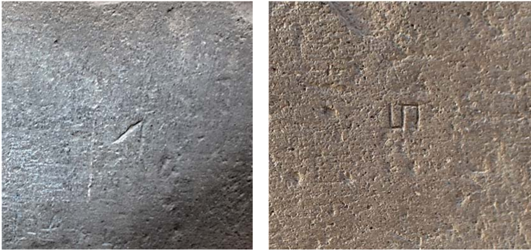
Figure 2-7: The grand mosque of al-Mahdiyya. Two examples of the marks possibly put by stone carvers in the carving workshops. Photo credit: Author.
