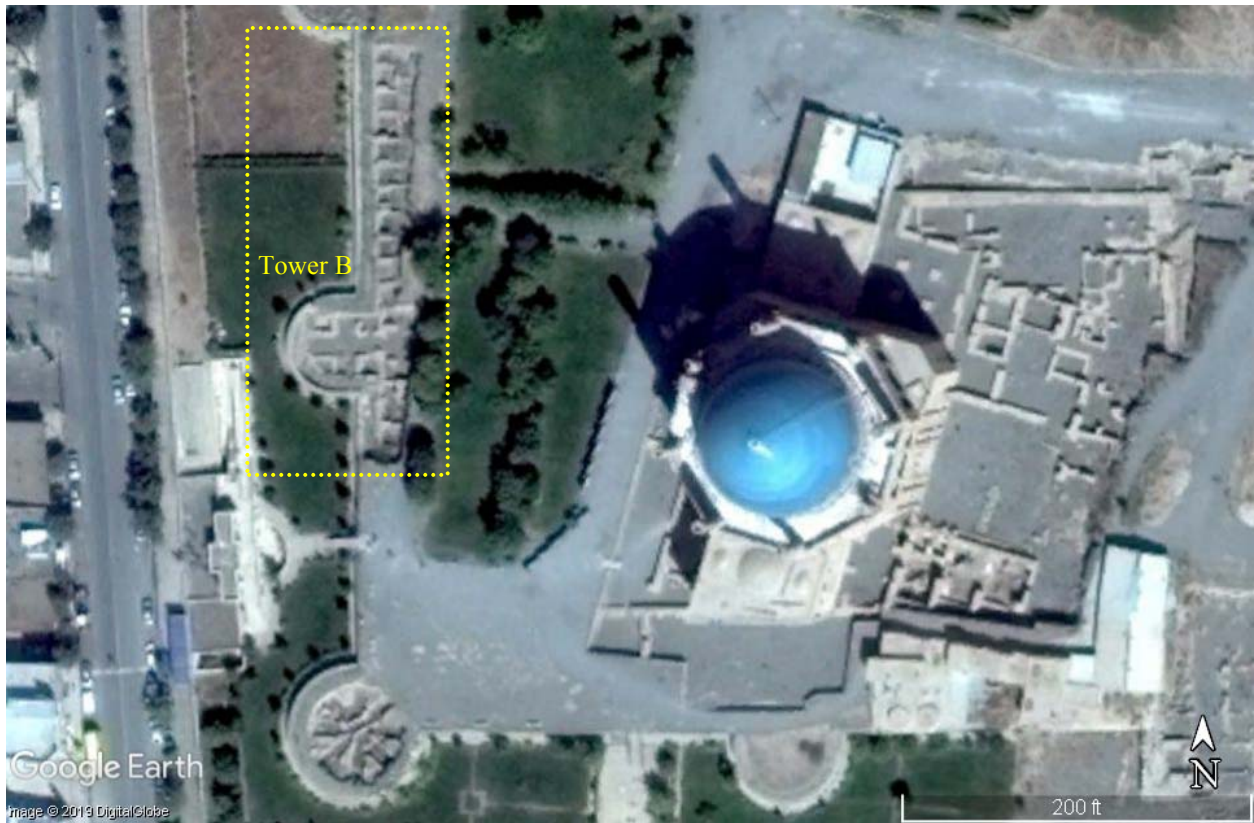
Figure 3-8: The row of cells built along the wall and the room built inside tower B with a cruciform layout. Photo credit: Google Earth. 2019 DigitalGlobe. Imagery date: 9/19/2014.
