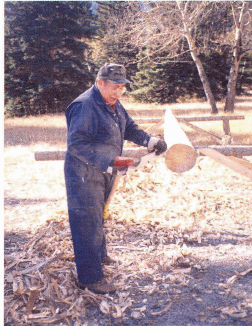
Figure 6.4 - Mike Moberly hewing replacement beams for the main structure of the Ewan Moberly Homestead. Source: Parks Canada Agency ID#283R-mh0102.
