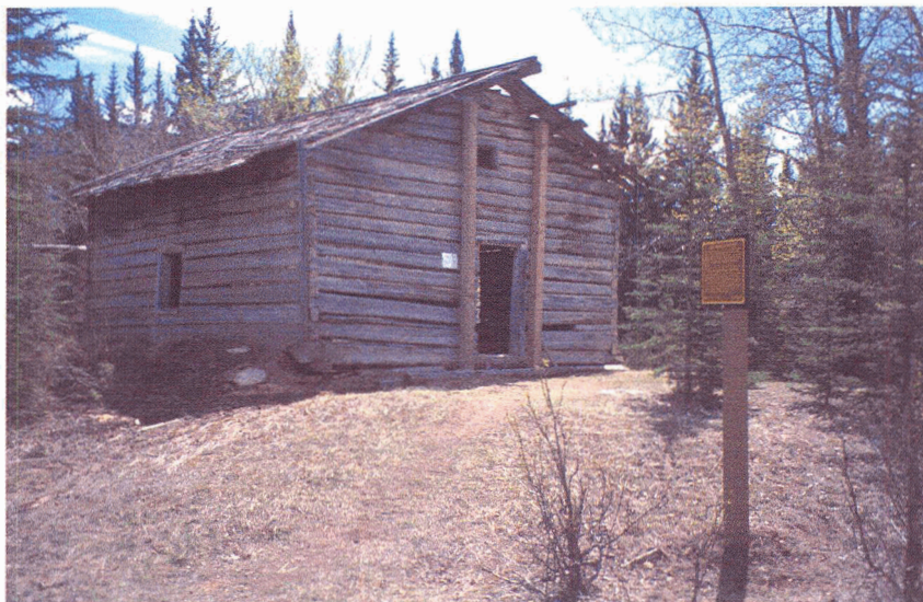
Figure 6.5 - Stabilizing the EMH main building in preparation for restoration (photo orientation: eastward facing). Source: Parks Canada Agency ID#283R-mh0018.
