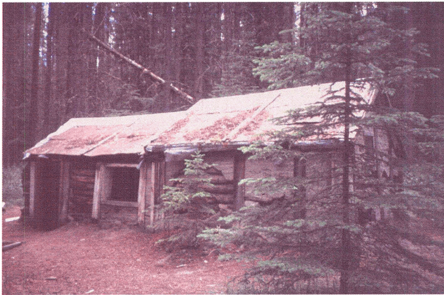
Figure 6.11 - Billy Carver Cabin, BNP (photo orientation: eastward facing). Photo: July 2001.
