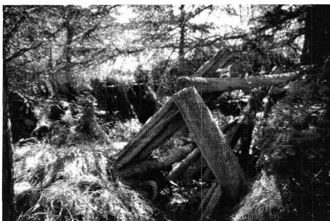
Figure A.14 - Edna Lake Structure (photo orientation: northeastward facing). Photo: July 2001.
