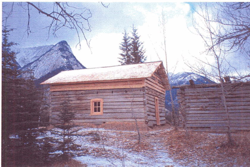
Figure 6.7 - Ewan Moberly Homestead: post stabilization (photo orientation: westward facing). Source: Parks Canada Agency ID#283R-mh0089.
