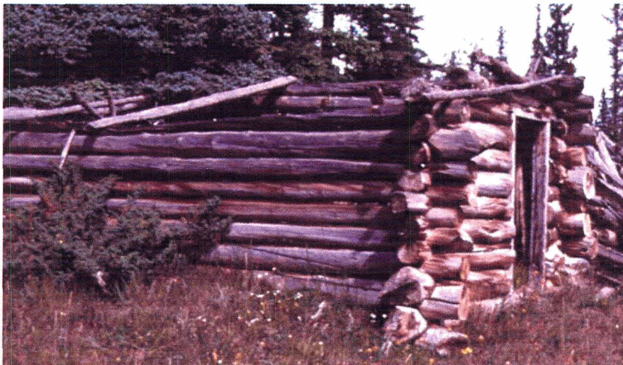
Figure 2.2 - Celestine Lake Road Railroad Construction Camp structure 3 (99P3). Source: Smith 1999.
