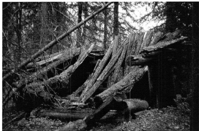
Figure A.54 - Fatigue Creek Cabin (backside view) (photo orientation: southward facing). Photo: July 2001.
