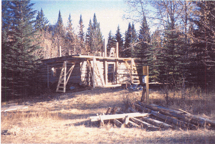
Figure 6.6 - In progress: replacement of roof and associated features (photo orientation: eastward facing). Source: Parks Canada Agency ID#283R-mh0029.
