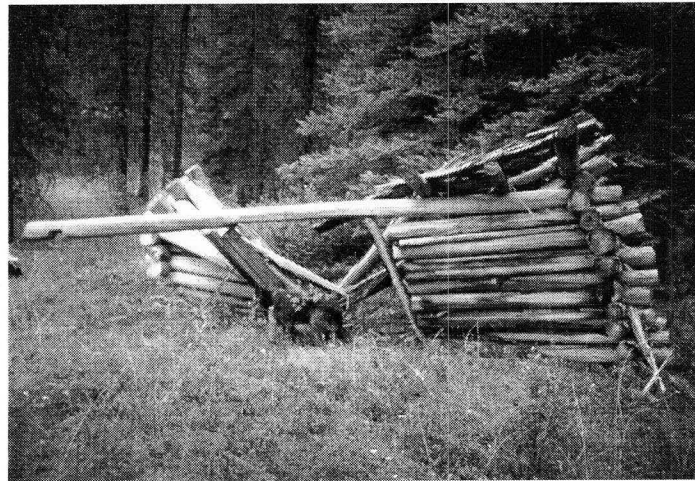
Figure A.56 - Kootenay River Cabin: front of section 1 (photo orientation: northward facing). Photo: July 2001.
