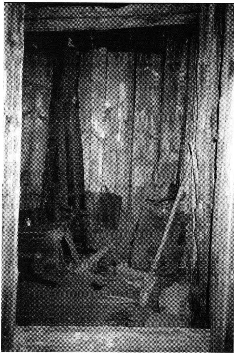
Figure A.50 - Bill Peyto Cabin interior: remnant materials. Photo: July 2001.
