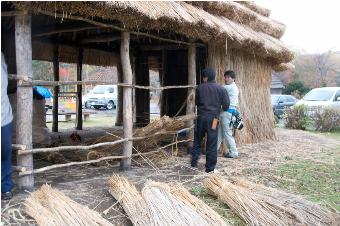
Figure 5 Two Ainu Workers Thatching the wall of a Cise on the Kotan Restoration Site
