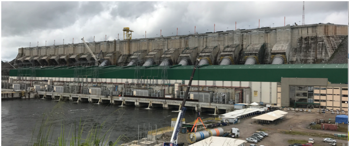
Figure 4: Belo Monte power plant. April 19, 2018. At that time, there were ten turbines installed and only three of them generating energy. Source: Author's personal files.
