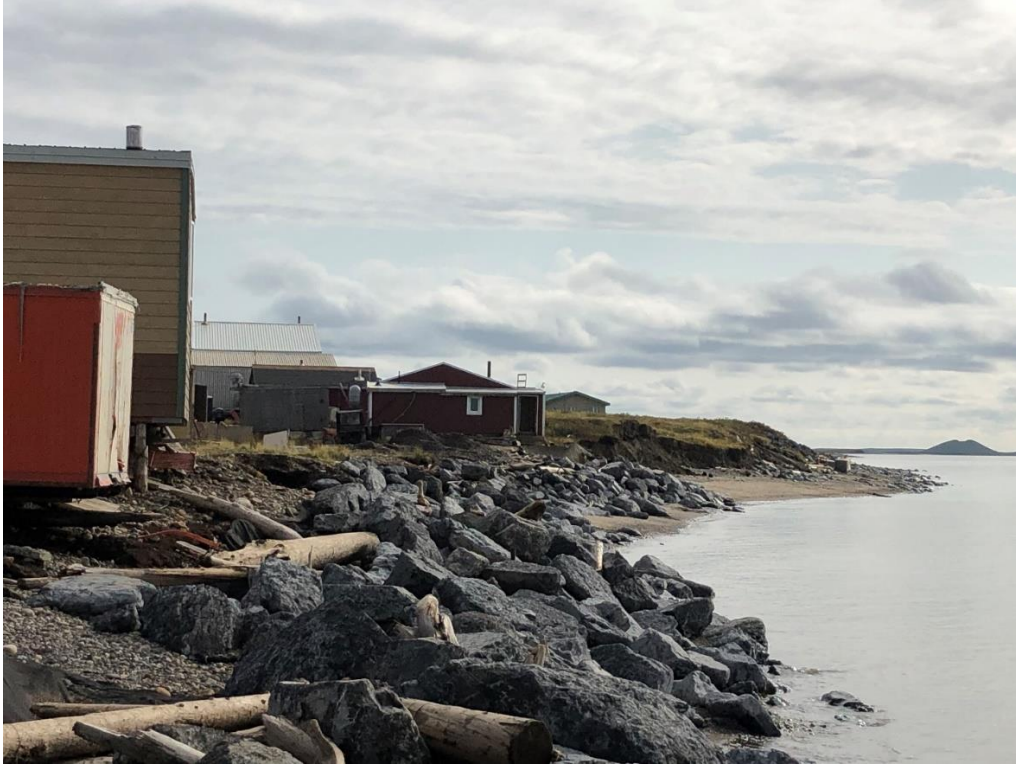
Figure 5. Homes in Tuk at risk due to erosion of the coastline, Aug. 2019. These homes were moved inland in 2020. You can see one of the prominent pingos in the background. Photographer: Letitia Pokiak.
