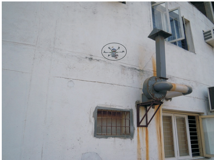
(a) Structural Inspectoin
