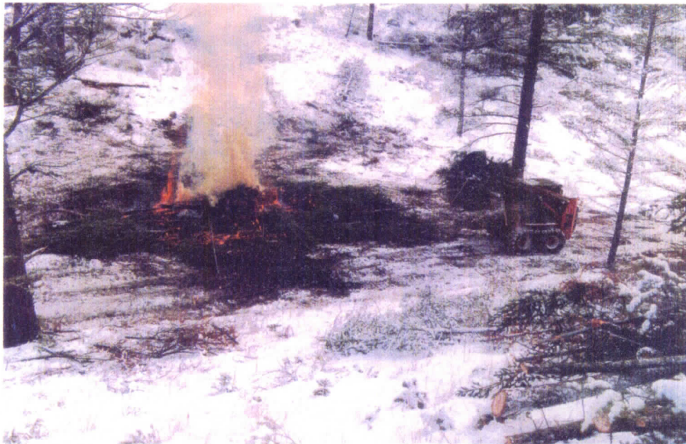
Figure 42: Front-end loader moving tree slash to sloop for burning at Stoddard Creek
