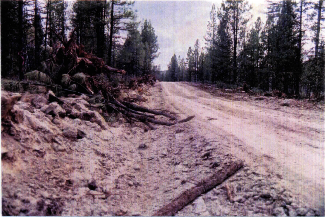
Figure 77: Condition of upgraded timber haul road bisecting Site DkPw-013, looking south
