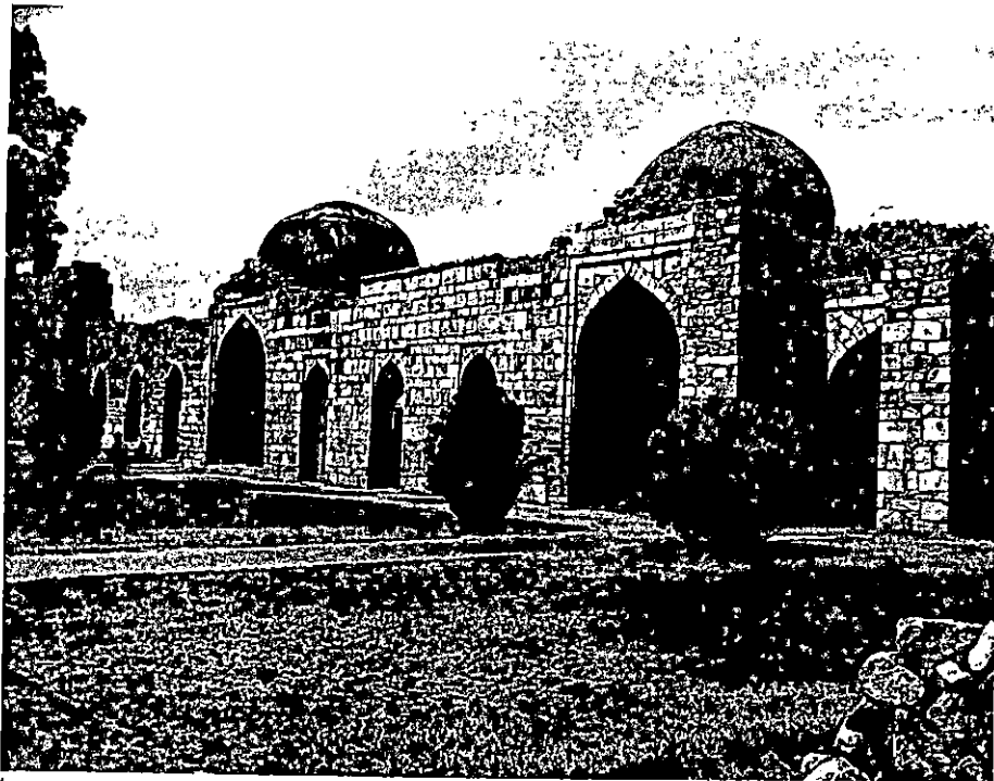
Plate XXVI. West Block Facade
