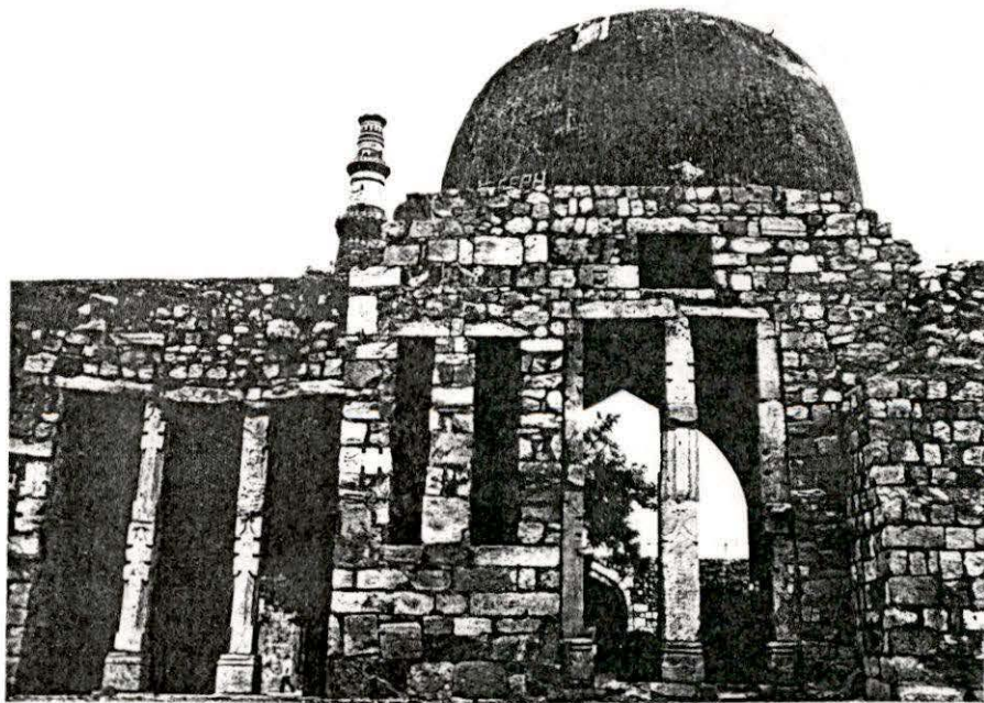
Plate XXVIII. West Block Exterior Wall (detail)
