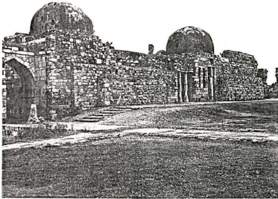
Plate XXVII. West Block Exterior Wall
