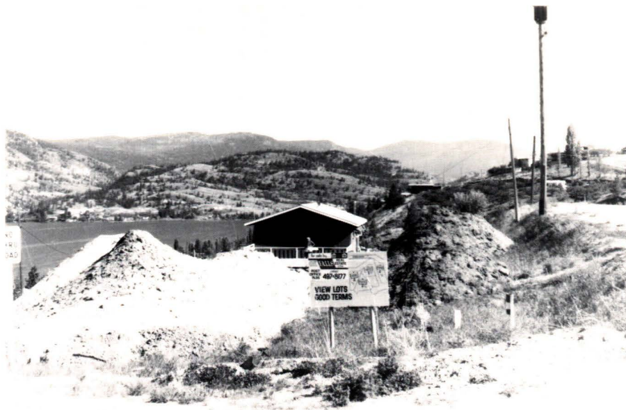
Plate 4. New home being constructed in a small subdivision at Kaleden.
