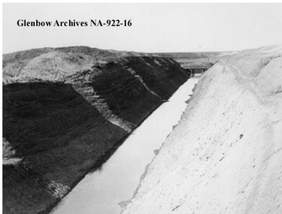
Figure 2: The Pot Hole Creek Diversion Canal outside of Magrath, Alberta, constructed largely by LDS settlers and missionaries (Unknown 1900).
