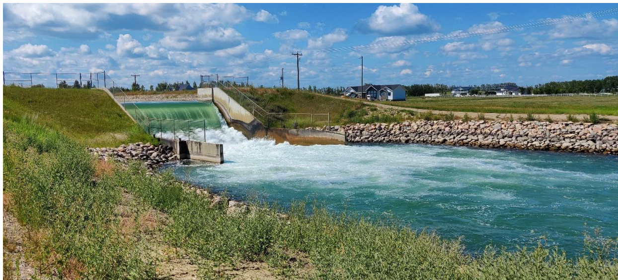
Figure 3: An irrigation canal located outside of Raymond, Alberta. The contemporary iteration of a canal system originally constructed by LDS settlers and missionaries (C. W. Campbell 2022b)
