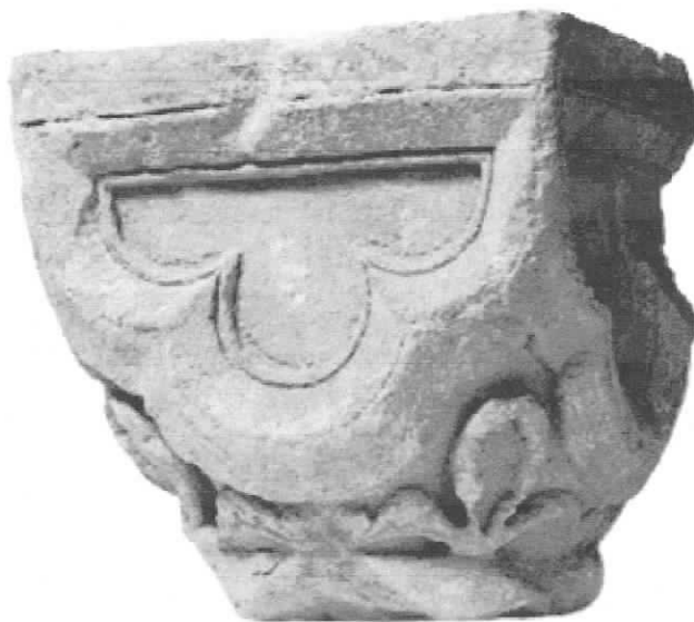
Fig. 23 Winchester Cathedral, triforium gallery, column capital showing sunken trefoil, c. 1150
