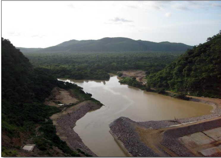
Figure 8: River diversion during dam construction, 2009. Photo by Ann Stahl
