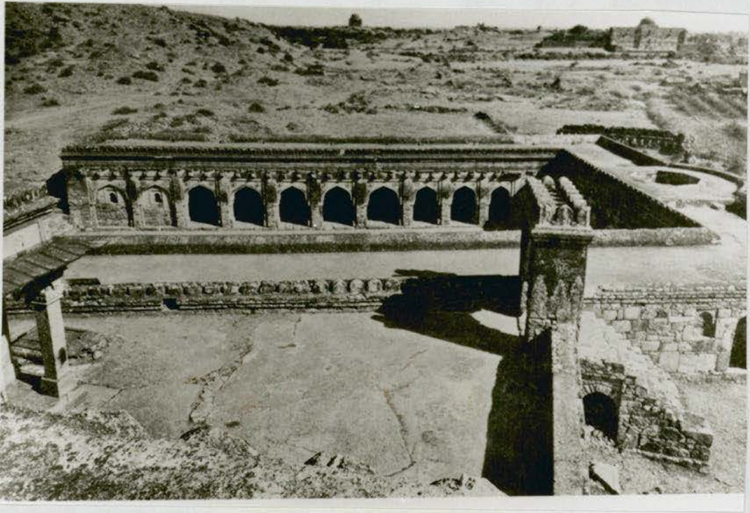
Figure 23 Rajon-ki Baoli - view of tank
