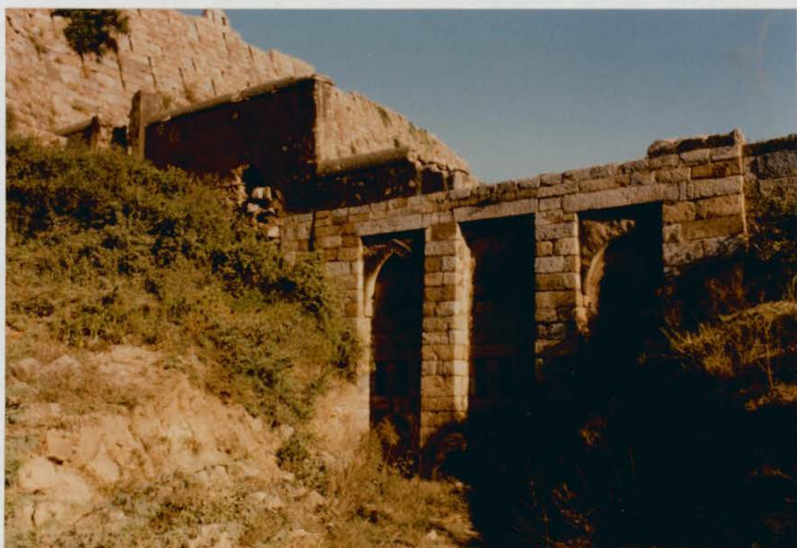
Figure 61 Sluice gate - south wall of Tughluqabad
