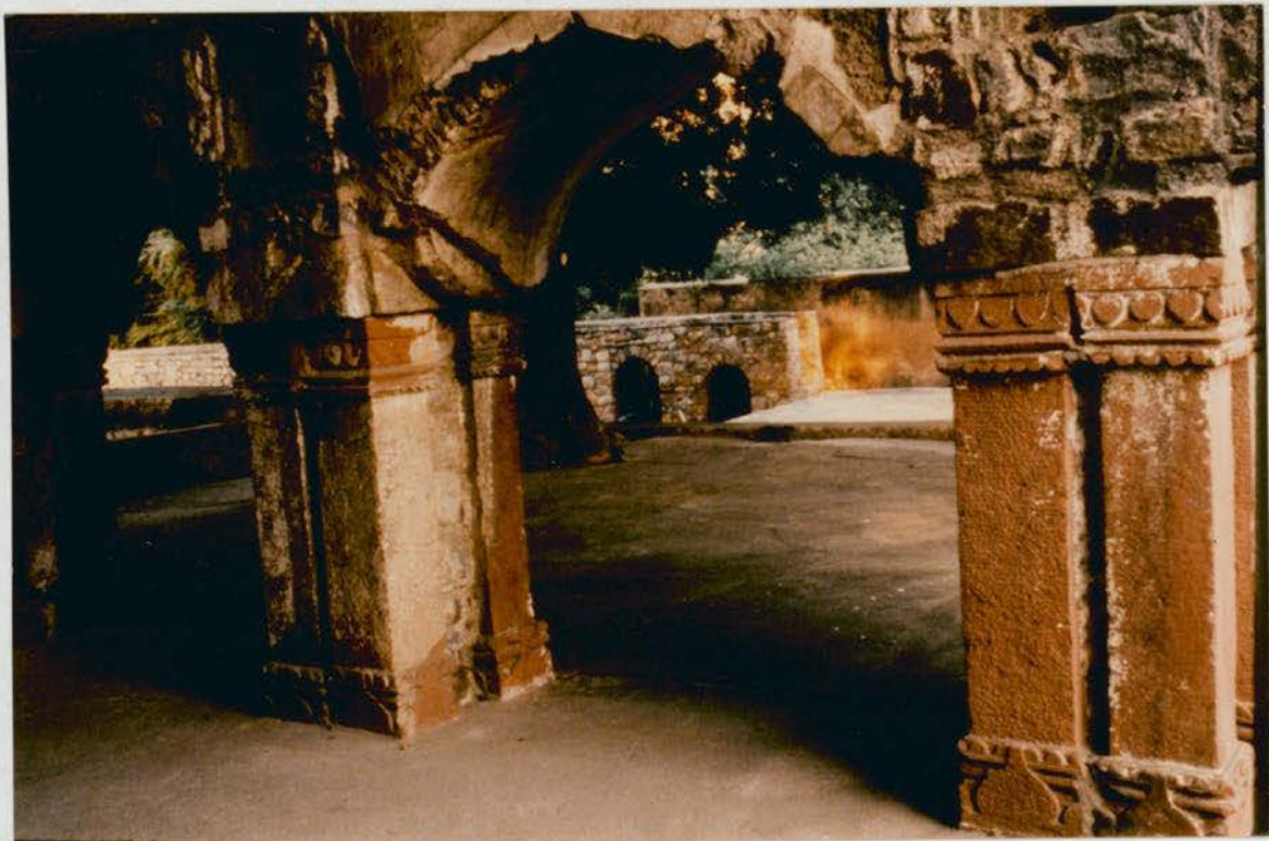
Figure 45 Ugrasen-ki Baoli - south end - mosque pillars
