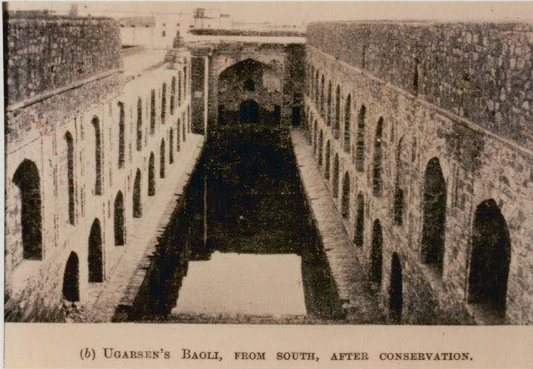
Figure 39 Ugrasen-ki Baoli - c.1926 - after repairs
