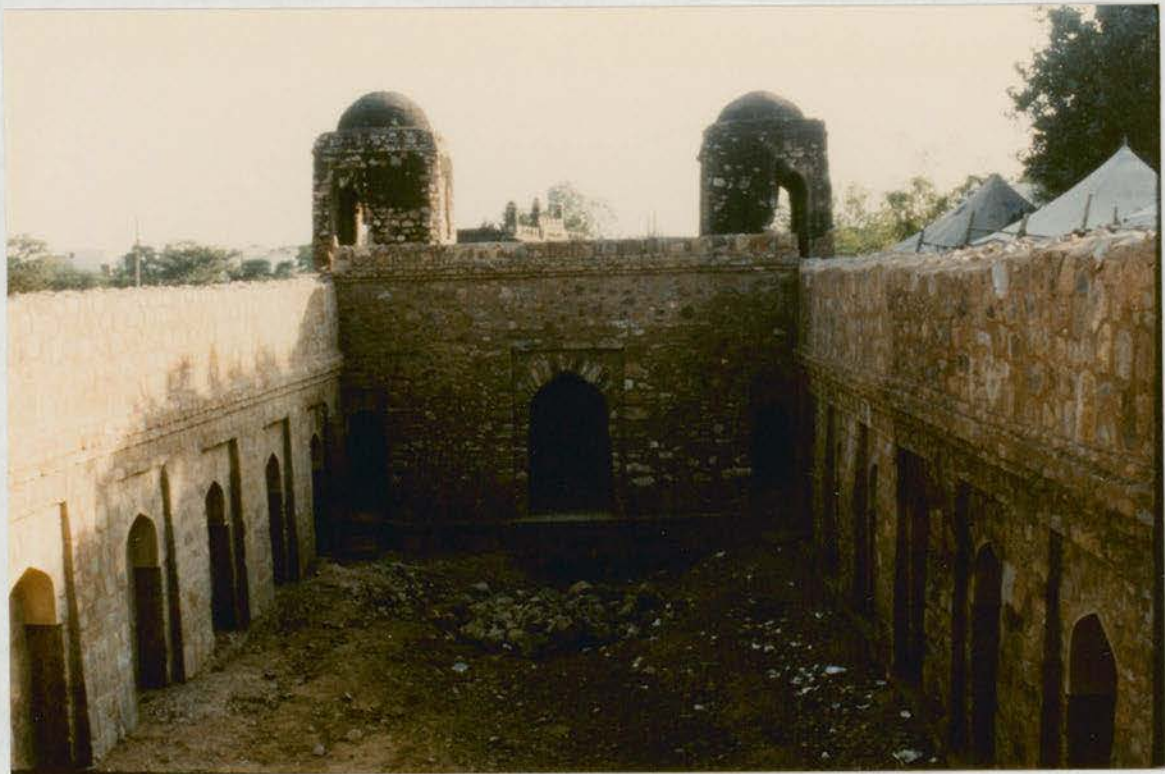
Figure 48 Baoli south of Wazirapur ka gumbad - south - recent repairs
