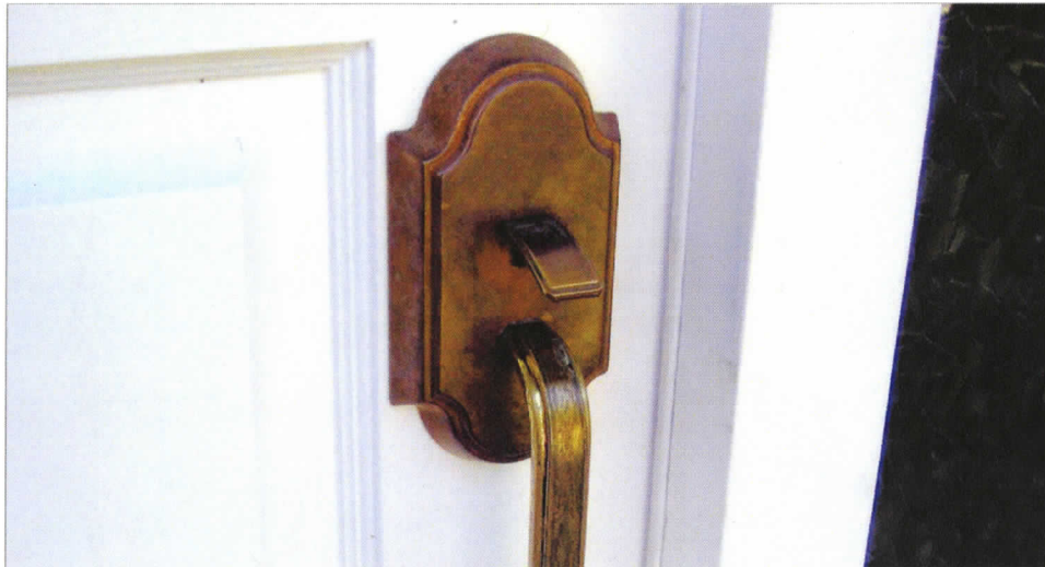
Figure 4.1: An example of social convention and aesthetics overruling usability. The design of a typical entry way door handle affords two actions: pushing down on the button and pulling. Unfortunately, the front door of most homes always open inward and the ergonomics of the handle makes pushing awkward.
