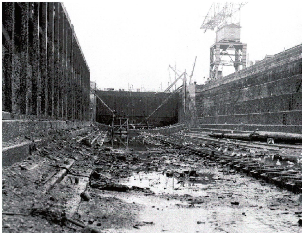
FIRST GRAVING DOCK PUMPED OUT FOR REHABILITATION, 1945
