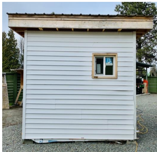
Figure 5.1 The experimental structure, showing the wall considered for analysis
