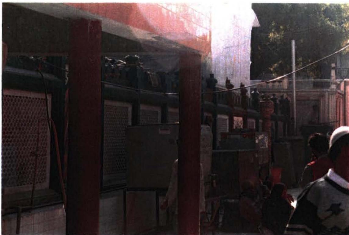
Figure 55: Photograph showing post and beams of original enclosure on east side of the dargah . December 1998. 257
