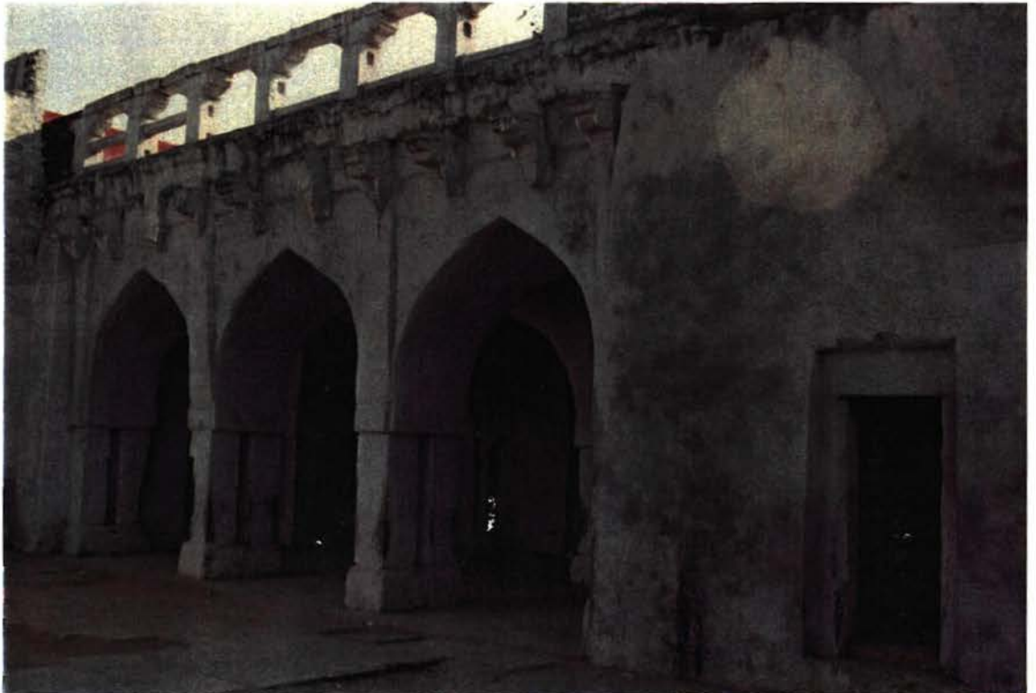
Figure 28: Photograph of unidentified building at Mahihpalpur, Delhi, resembling chillagah . December 1998.
