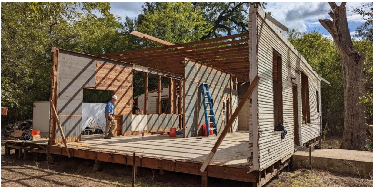
Figure 5. Students in Material Innovation Center Learning Building Deconstruction
