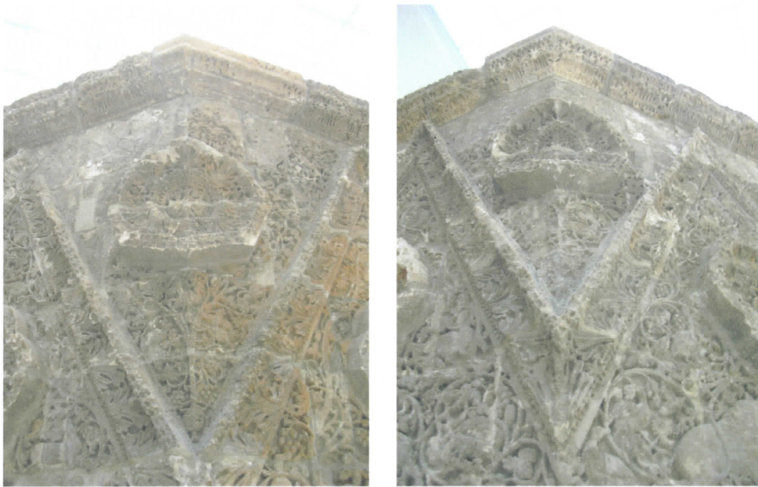
Figure 91 Rosettes in obtuse spaces, Mshatta façade.
