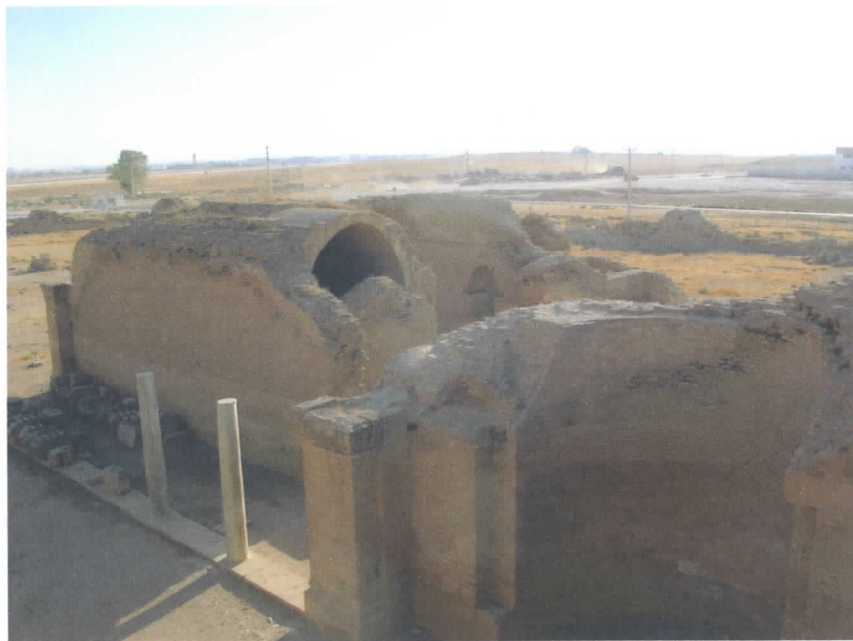
Figure 79 View of the brick walls of the audience hall, Mshatta.
