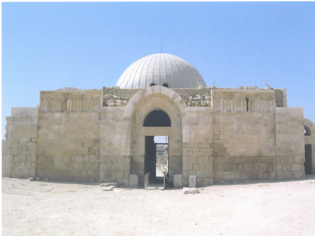
Figure 28 Reception hall of the Umayyad palace at the Citadel of 'Amman, with reconstructed dome.
