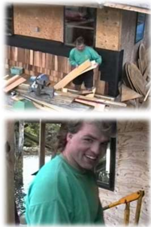
Figure 142 - Shaun Shelongosky in the midst of finishing the construction of the Ark Café and Bed & Breakfast, early 1990s.
