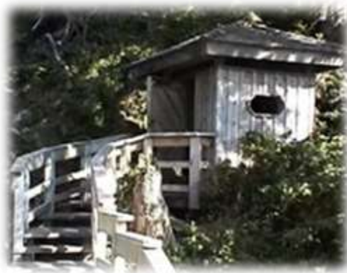
Figure 158 - The original changing shelter, built during the construction of the new boardwalk in the 1990s.
