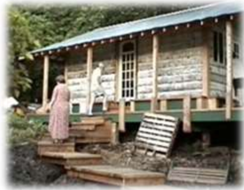
Figure 162 - Dick Woodsworth’s cabin at the foot of the Springs-side dock, rebuilt in the late 1990s. In the late 2000s, it would be rented for many years to serve as accommodations for the Park Facility Operators.
