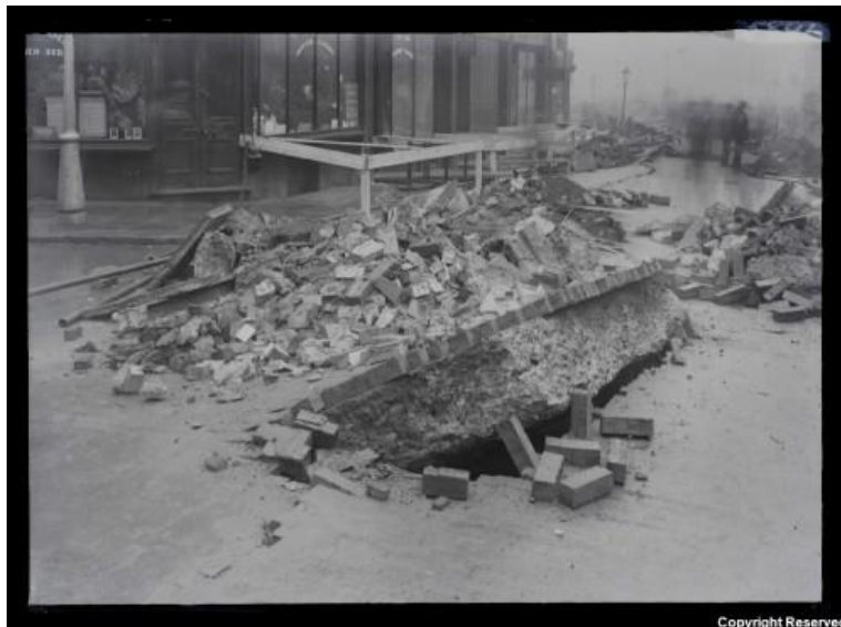
Figure 5 Holborn gas explosion, 1928, https://www.ianvisits.co.uk/blog/2013/12/20/1928-a-massive-gas-explosion-rips-along-holborn/
