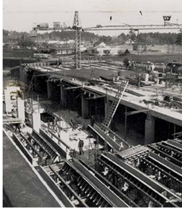
Library addition under construction, 1972. ▲
