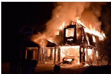
Figure 1 Residential Structure Fire
