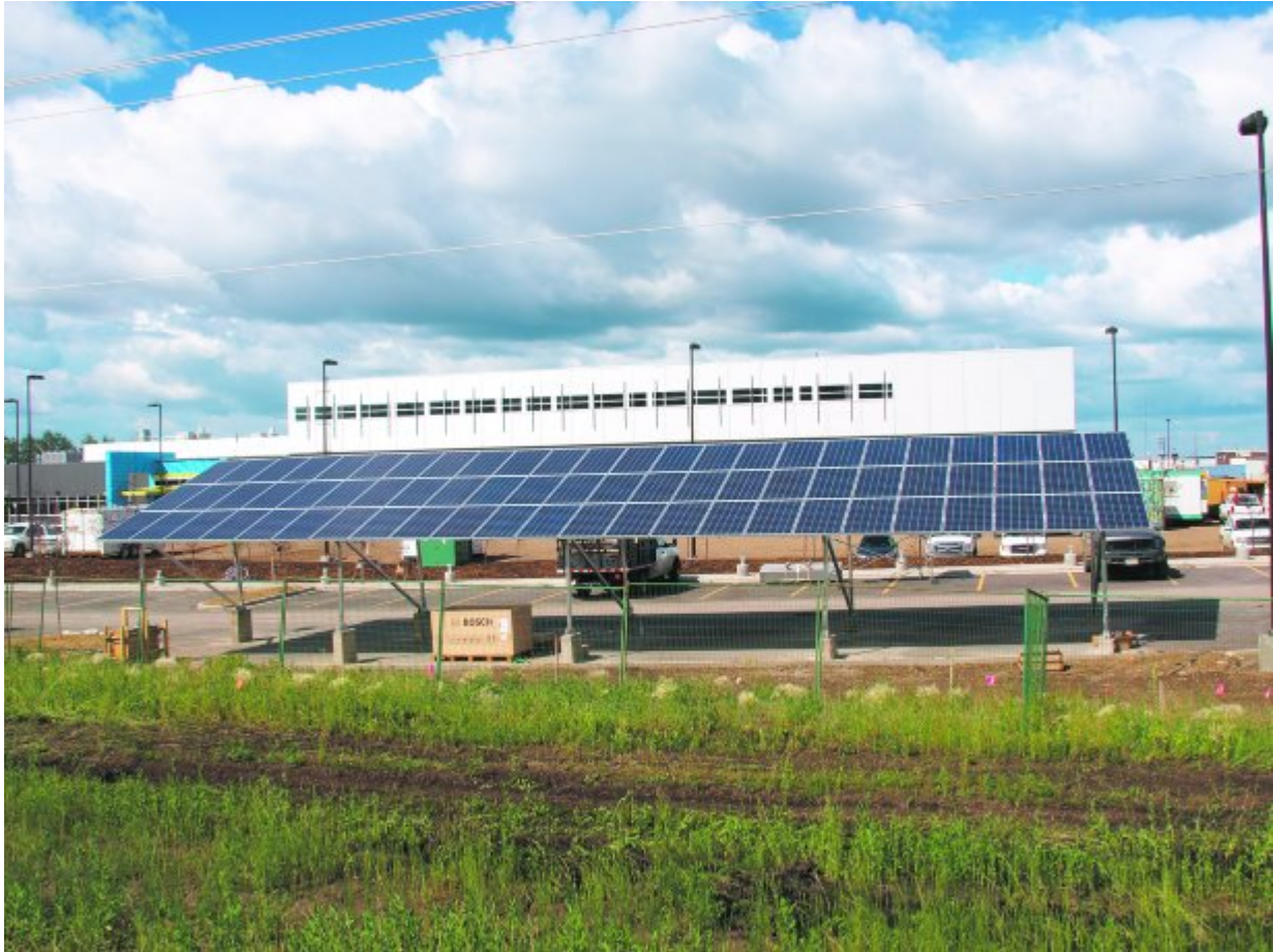
Figure B2. A solar carport installation at the new regional Public Operations Centre, constructed in 2014 for the Regional Municipality of Wood Buffalo in Northern Alberta (Christian, 2014, Figure 1).
