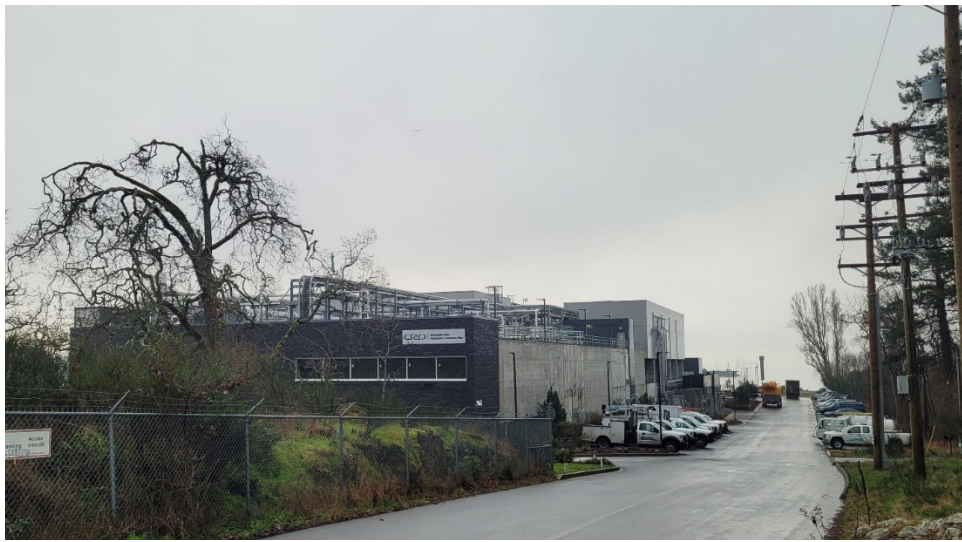
Figure 26: Site photo of WWTP3.
