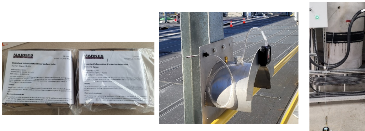
Figure 11: (Left) Photo of Sorbent tubes in package from Markes International. (Mid) Photo of sorbent tube deployed at WWTP collecting ambient air around primary treatment. (Right) Photo of sorbent tube deployed into ductwork.
